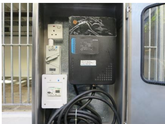
7 kW, single phase AC charger
