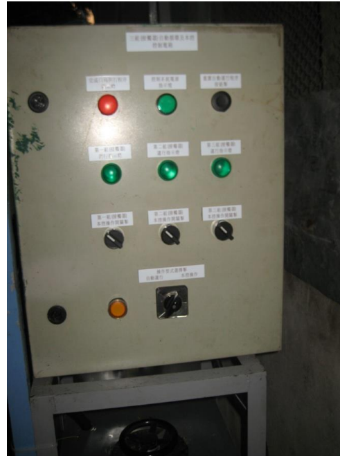
Photo 4.6. PLC controller for load bank
