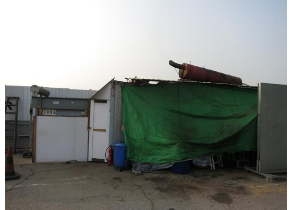
Photo4.10. Remote radiator and water scrubber
