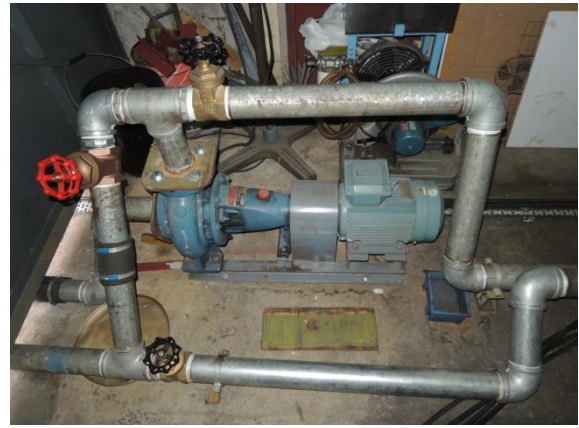
Photo 4.4. Water pump for engine cooling
