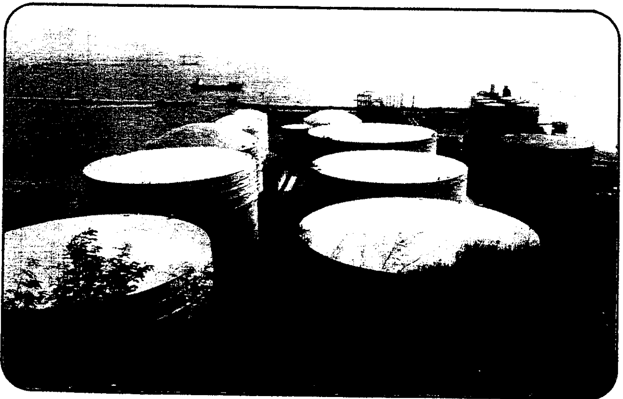
The Oil Depot at Tsing Yi Island
