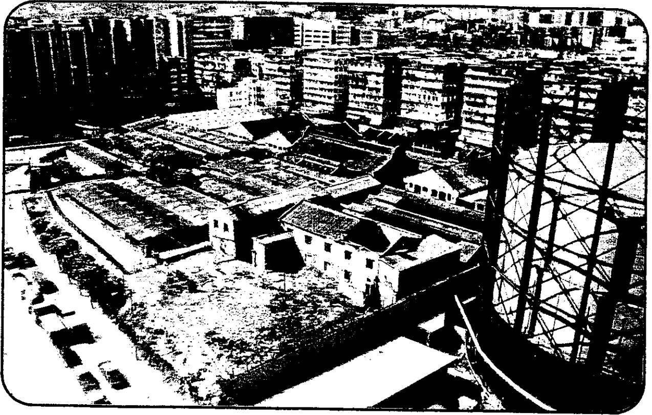
The Ma Tau Kok gas plant incompatibly situated in an urban area
