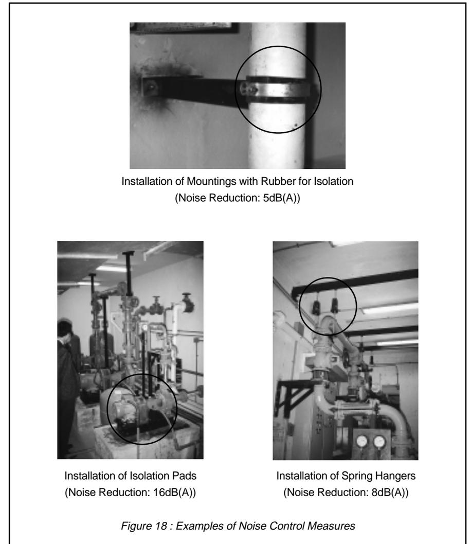
*Figure 18 : Examples of Noise Control Measures*
