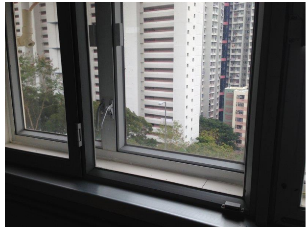
Figure 6: Secondary Glazing Window
