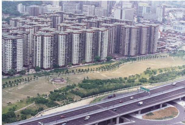
West Kowloon Expressway was planned to separate from Mei Foo Sun Chuen by 150m landscape buffer. 3m high barriers were erected to reduce noise at Mei Foo Sun Chuen to meet the standard
