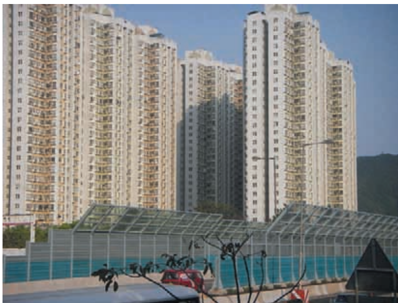
Retrofitting barriers at Fanling Highway
