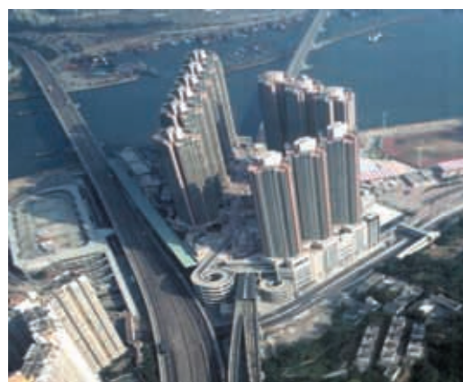
Barrier extended from podium and other measures included at the planning of Tierra Verde, Tsing Yi
