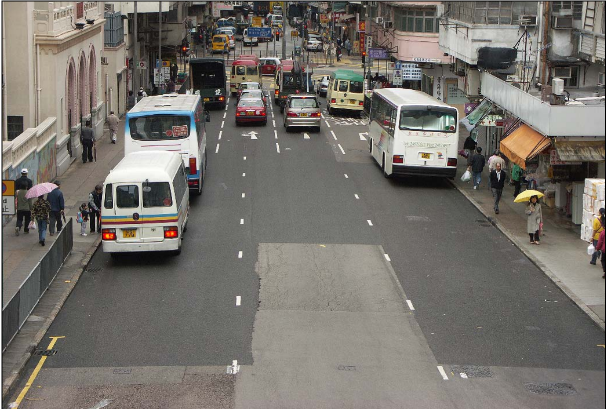
Fig. 51. Very short and busy road section on Shek Kip Mei Street with PMFC. LNRS would not be effective on such short section and with this type of traffic.
