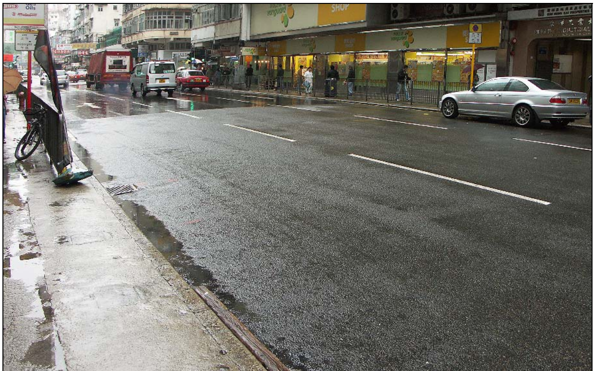
Fig. 54. PMFC on Un Chau Street appears to be totally saturated with water during moderate rainfall, and kerbside drainage is poor. No noise reduction could be heard.
