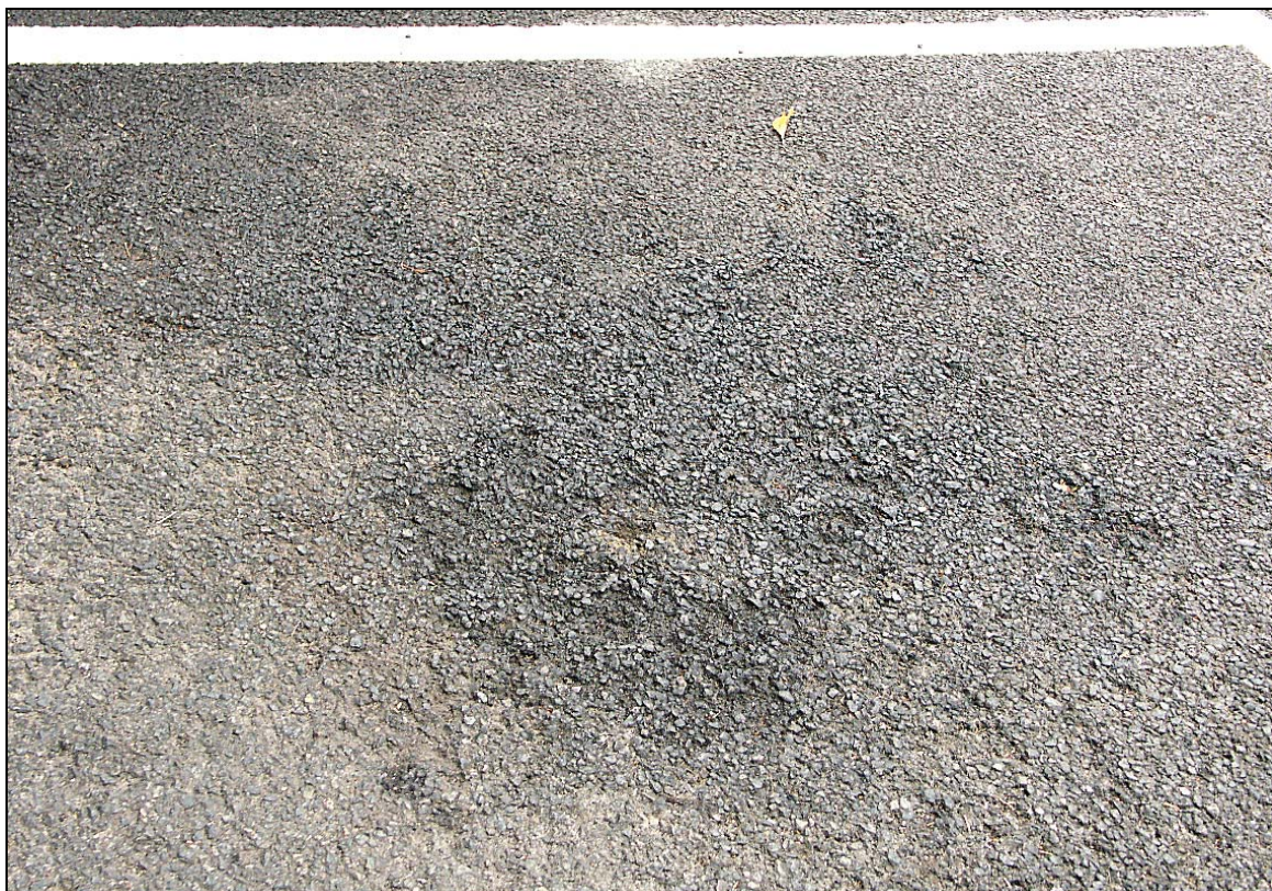
Fig. 34. Serious ravelling and clogging (lower left) in parking lane on Hing Wah Street.
