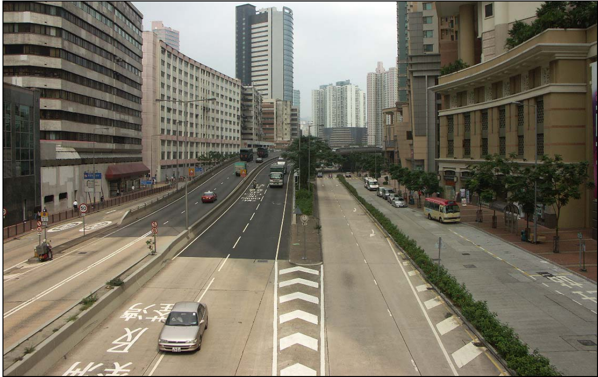
Fig. 39. Resurfacing with PMFC planned for the rightmost local street (close to mall at right) but should instead be made on the BRRC surface on the main road (Lai Chi Kok Road)
