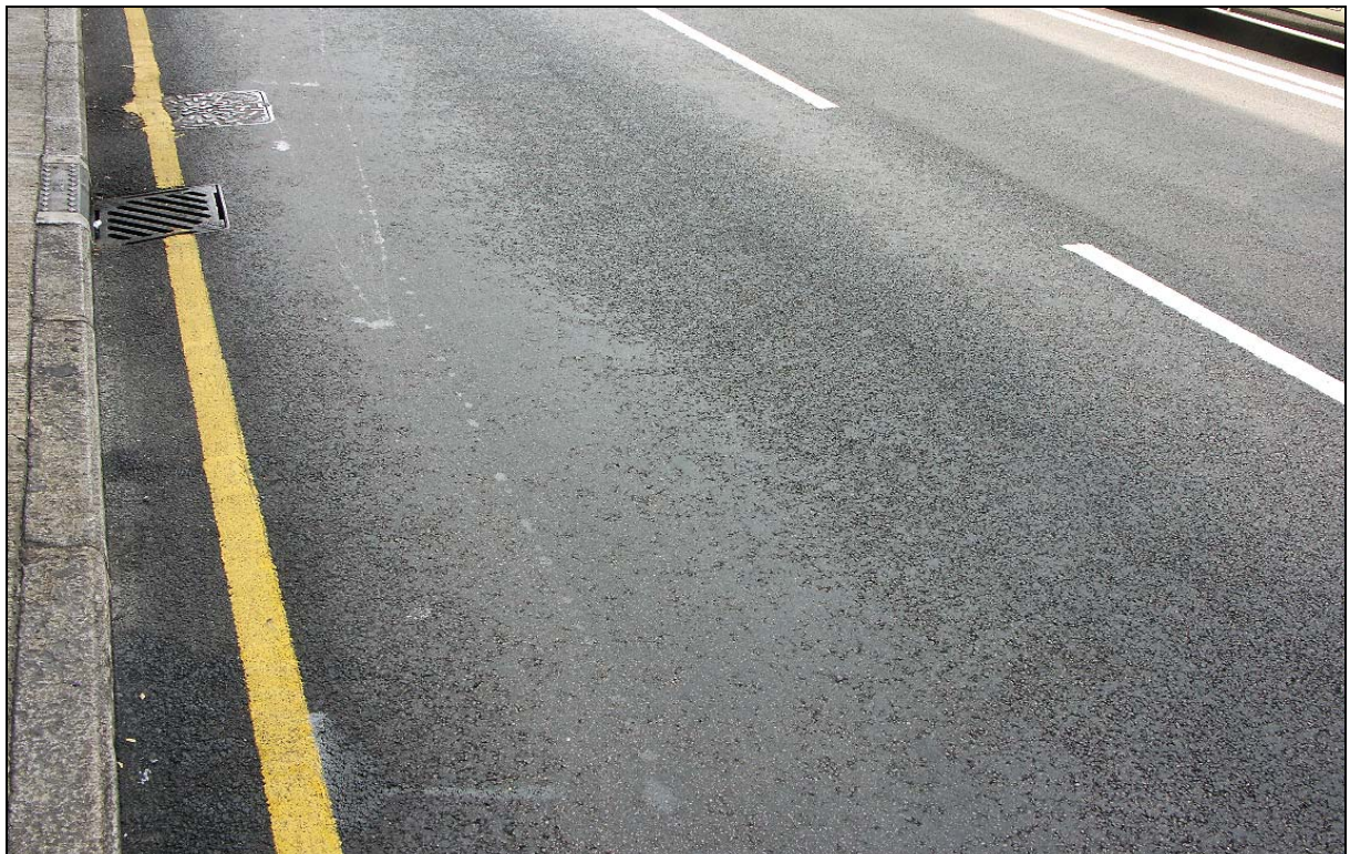
Fig. 38. SMA surface on Junction Road, flushing in left wheel track.
