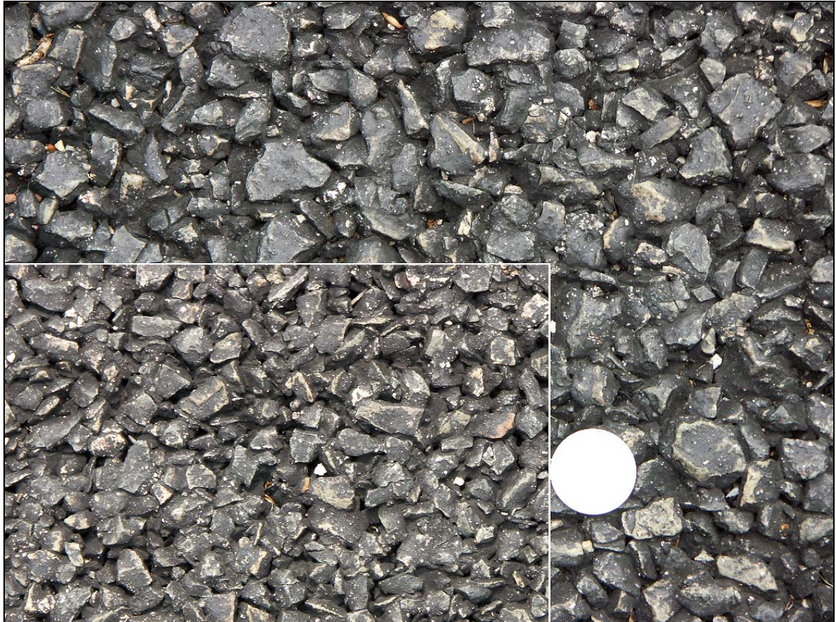
Fig. 37. PMFC on Chui Tin Street with max 20 mm aggregate, and with photo of 10 mm aggregate version inserted to scale. Coin is HK$ 1. Surfaces 9 months old, perfect condition.
