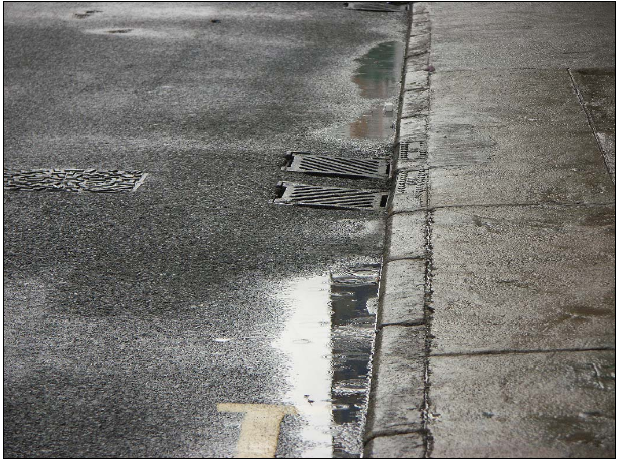
Fig. 53. Inefficient drainage at the kerb on Un Chau Street, potentially speeding up clogging.
