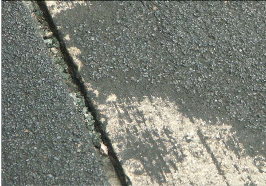
Fig. 4. Sho-bond surface dressing laid on BRCC slabs; close-up of surface with some damages (Lai Chi Kok Road). The underlying BRCC texture is seen in the lower right corner.
