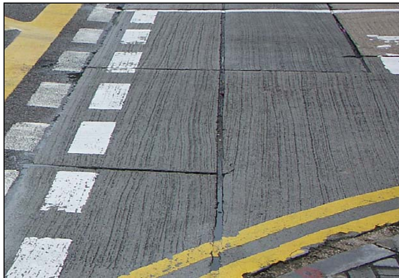
Fig. 2. Close-up of brushed cement concrete slabs. This is sometimes the type of surface being repaved with PMFC to reduce noise (Lomond Road intersection).
