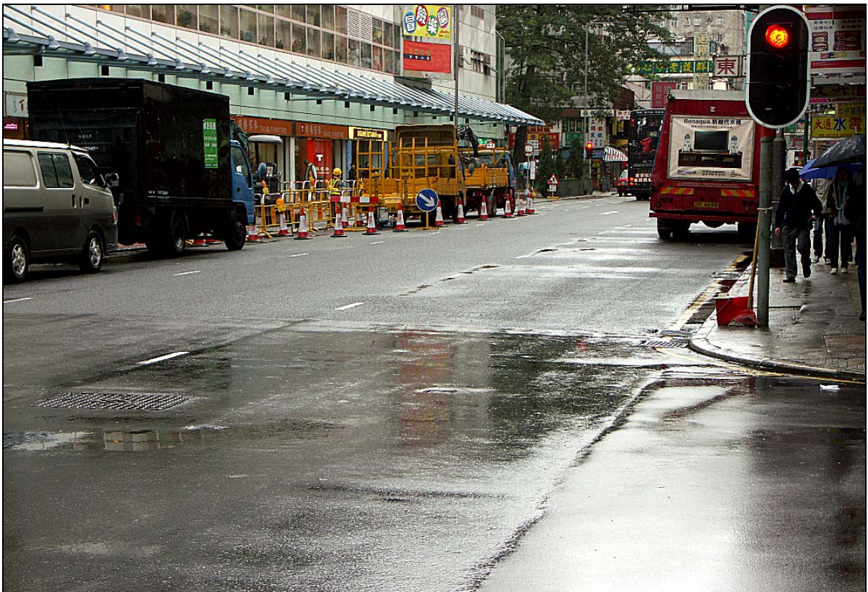
Fig. 52. Differences between dense asphalt and PMFC, also showing inhomogeneities in PMFC (right lane) probably caused during paving.
