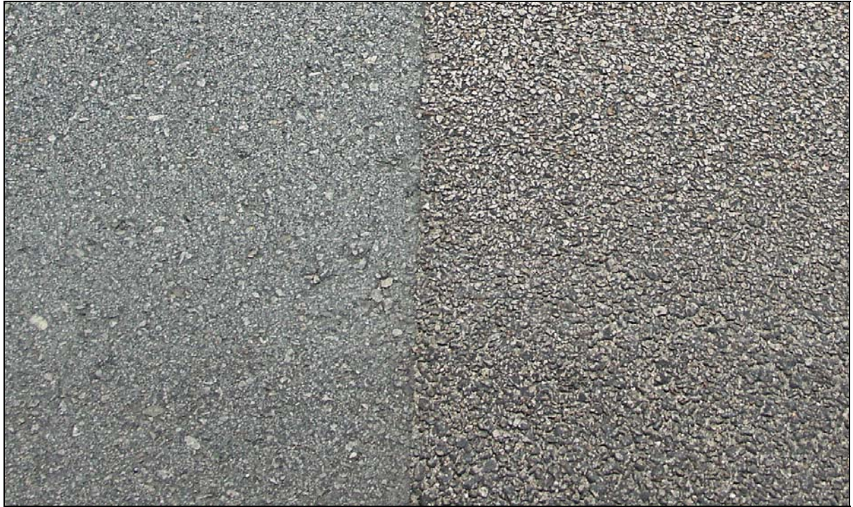
Fig. 27. Conventional DAC at left and clogged PMFC at right, both probably having 10 mm max. aggregate size but with some oversized chippings. Northwestern corner of Victoria Park.
