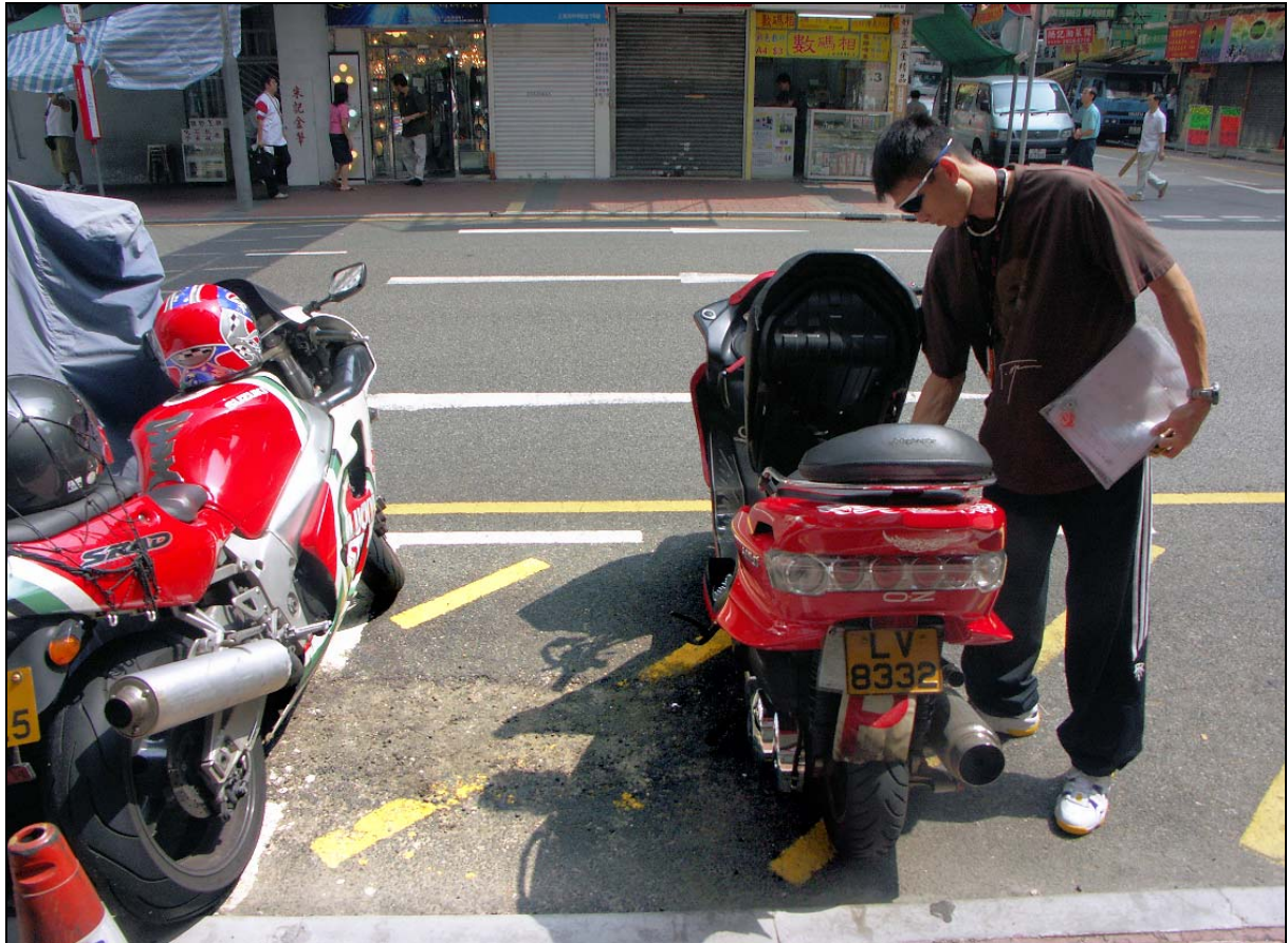
Fig. 47. Approx. 15 months old PMFC totally damaged (topmost chippings stripped off) by motorcycle stands on Shanghai Street. Surface also clogged due to poor kerbside drainage.
