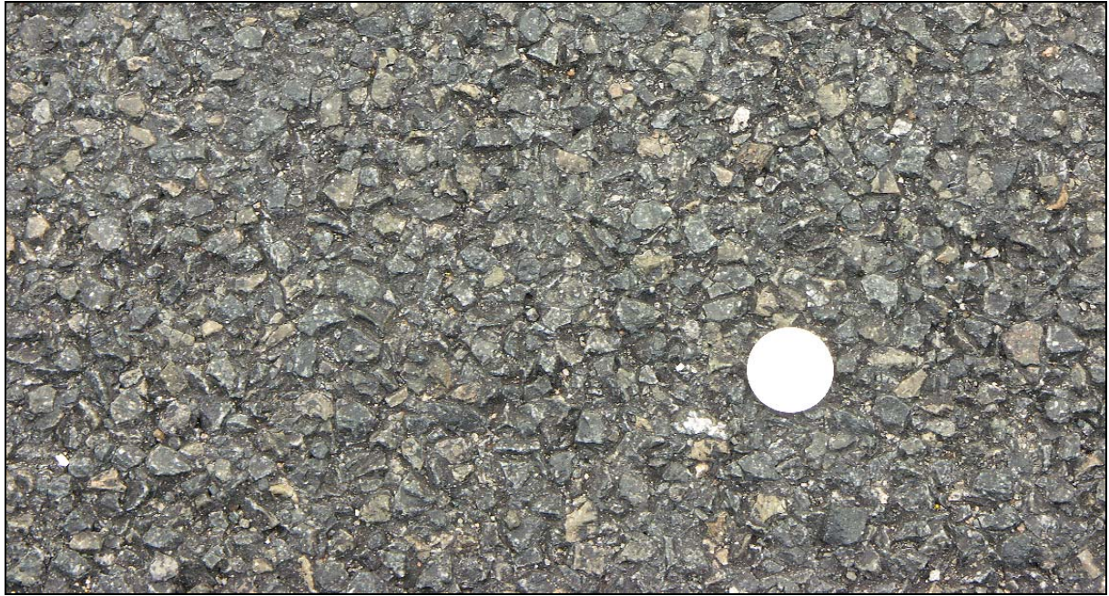
Fig. 45. Totally clogged PMFC, 3 years old, on Public Square Street. It looks like a surface dressing.
