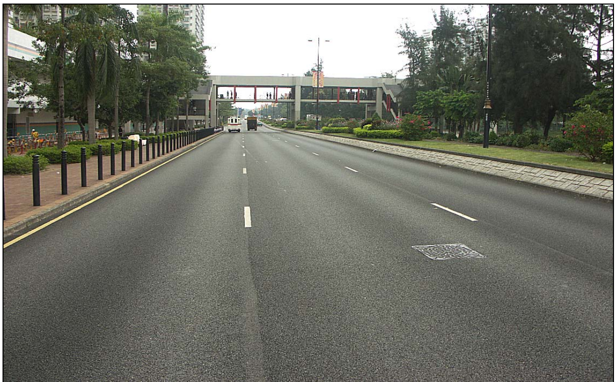
Fig. 48. Tai Po Tai Wo Road, posted speed limit 70 km/h, with 12 months old PMFC still in very good condition, despite no visible drainage at the kerb. Why manhole in the wheel track?
