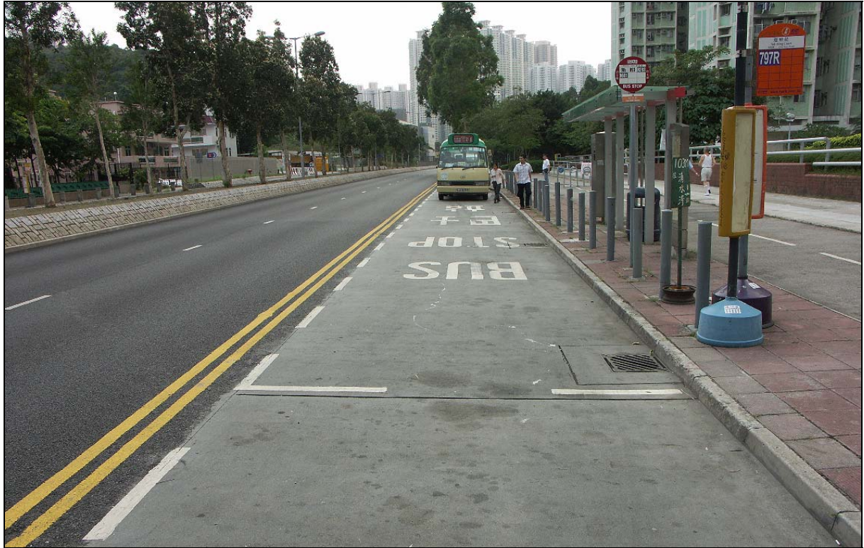
Fig. 35. Chiu Shun Road with 9 months old PMFC in perfect condition, and bus bay having stronger "Thin Bond Concrete" surfacing.
