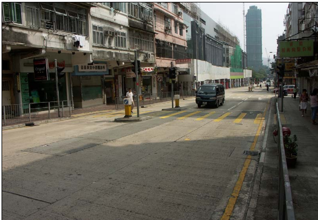
Fig. 1. Illustrations of a common brushed cement concrete (BRCC) surface on city street (Junction Road) often being the type of surface on which a PMFC is laid.
