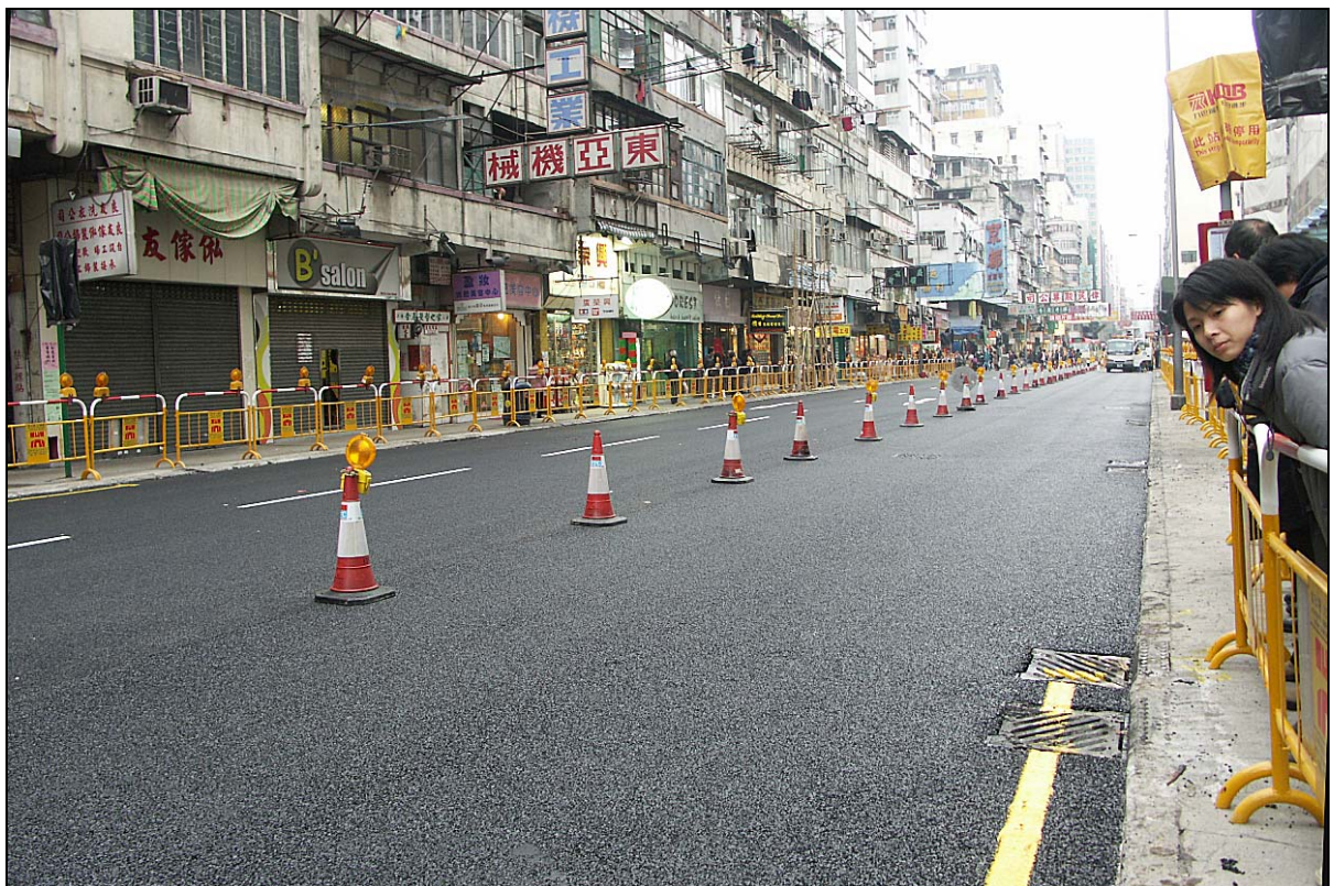
Fig. 32. Resurfacing with PMFC just finished on Un Chau Street. Note the location of gullies at the kerbside, with pair of gullies together but long distance between the pairs.
