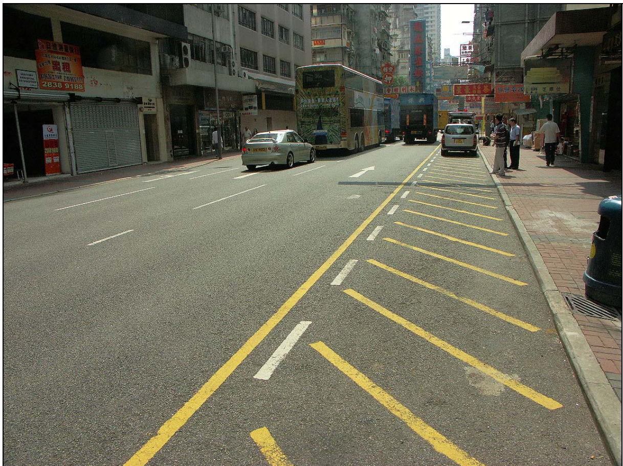
Fig. 46. Practically no drainage at the kerb on this approx. 15 months old PMFC on Shanghai Street. Some ravelling in rightmost lane, plus serious clogging along the entire kerb.
