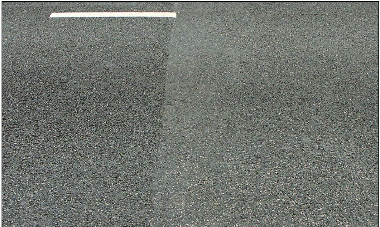
Fig. 36. Separation problem on Chiu Shun Road, due to binder having collected at the very bottom of a truck load during transportation from the asphalt plant.
