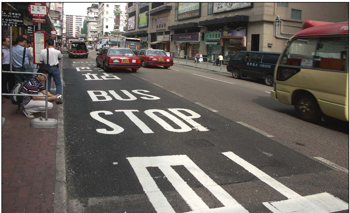
Fig. 42. Bus stop on Ma Tau Kok Street has been resurfaced due to damages by busses; despite the main area being resurfaced with PMFC only 10 months earlier.
