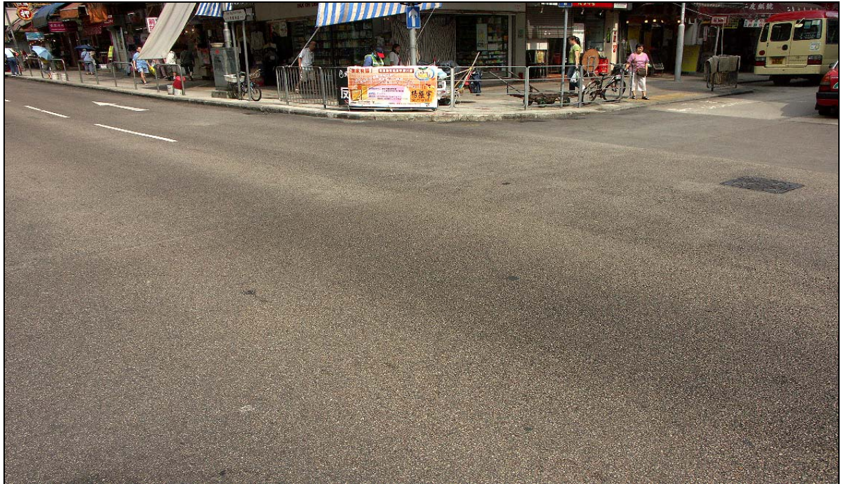
Fig. 43. Example of reasonably well working intersection with PMFC. Ma Tau Kok Street with 10 months old PMFC.
