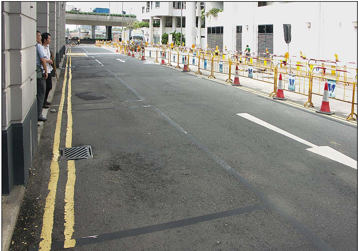
Fig. 44. Public Square Street with 3 years old PMFC, being seriously damaged in parking lane; perhaps aggravated by oil spillage. Roadwork in the other direction is not caused by PMFC problems.
