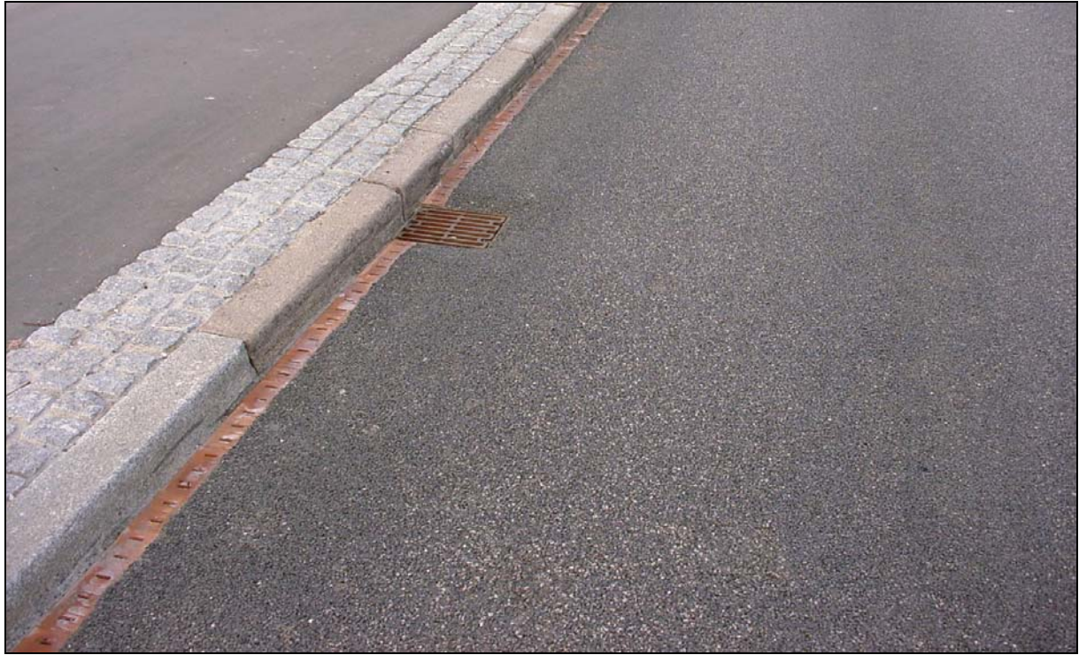
Fig. 21. Kerbside drainage system used in experiments with double-layer porous asphalt in the city of Copenhagen 1999-2006 (photo by the author).
