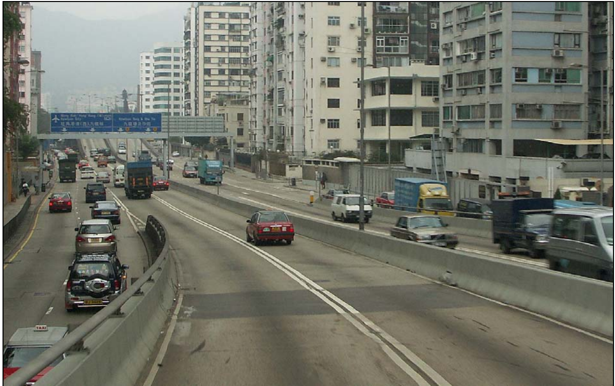
Fig. 29. PMFC on extremely demanding location (Princess Margareth's Road), approaching end of lifetime.
