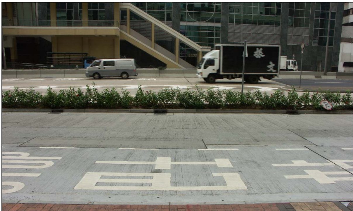
Fig. 61. Brushed cement concrete (BRCC) on Lai Chi Kok Road. Almost any dense bituminous surface with a texture depth of 0.5-1.0 mm will reduce noise in relation to this surface if tyre/road noise is substantial.
