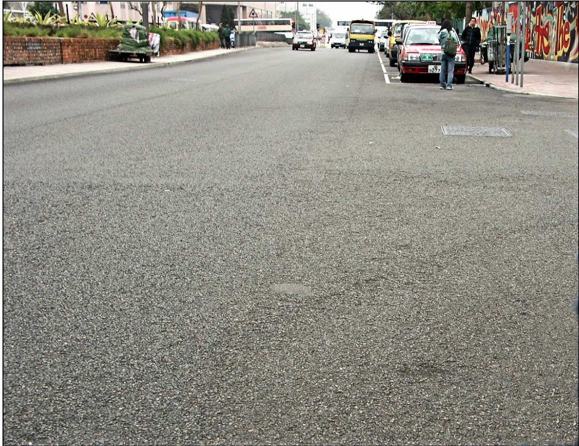
Fig. 33. Ravelling at intersection on Hing Wah Street, with one small spot being repaired.
