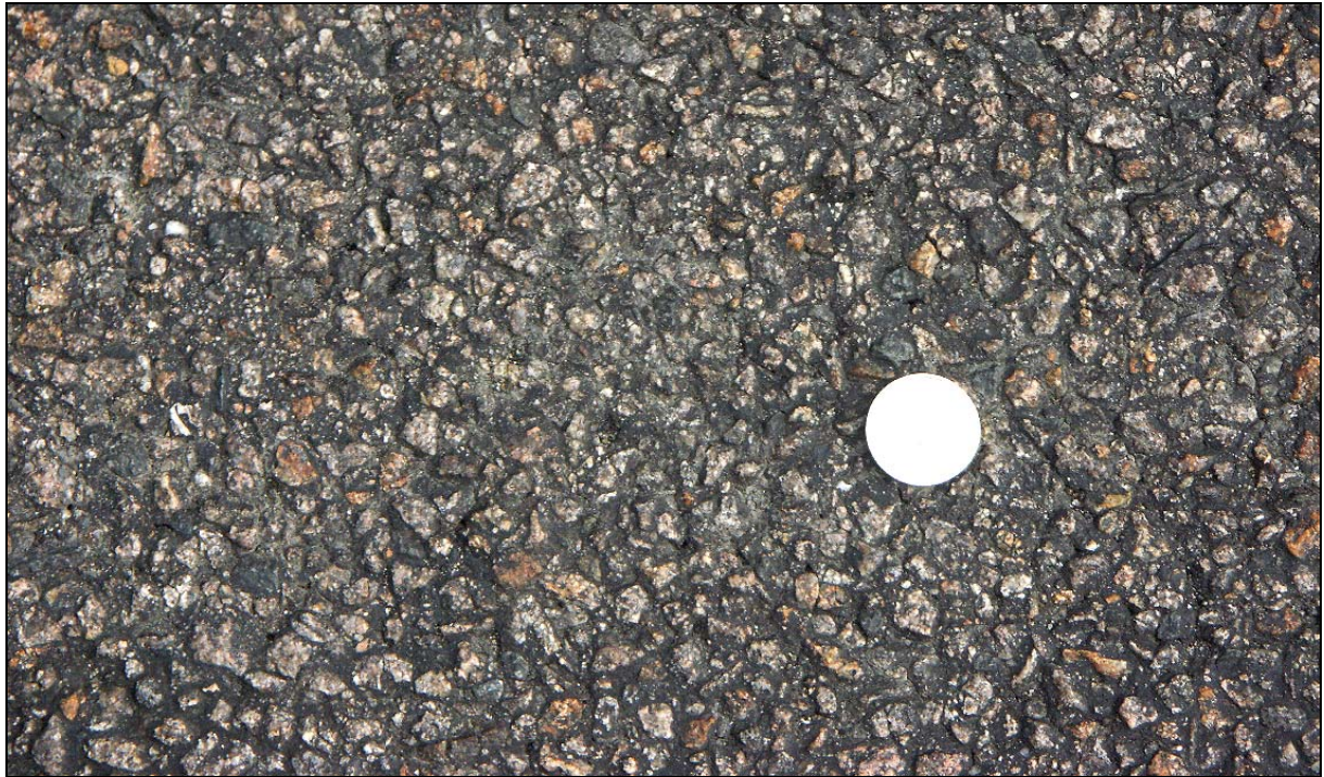
Fig. 41. Totally clogged PMFC on Ma Tau Kok Street, 0.5 m from the kerb. Coin is HK$ 1.
