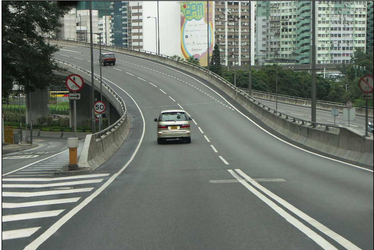
Fig. 49. Two months old PMFC on uphill section of high-speed road (Tseung Kwan O) with a significant gradient. The section had been repaved because of ravelling of old PMFC.
