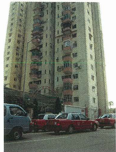
A general view of the "after" site
