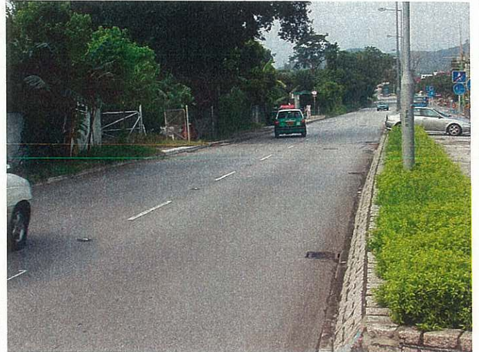
General view of the subjected road
