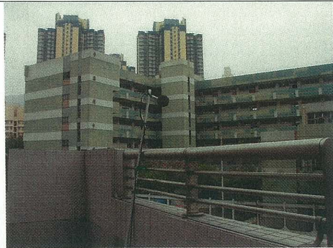
Measurement point at reference site ("after" site)
