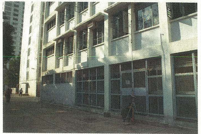
General view of the "after" site
