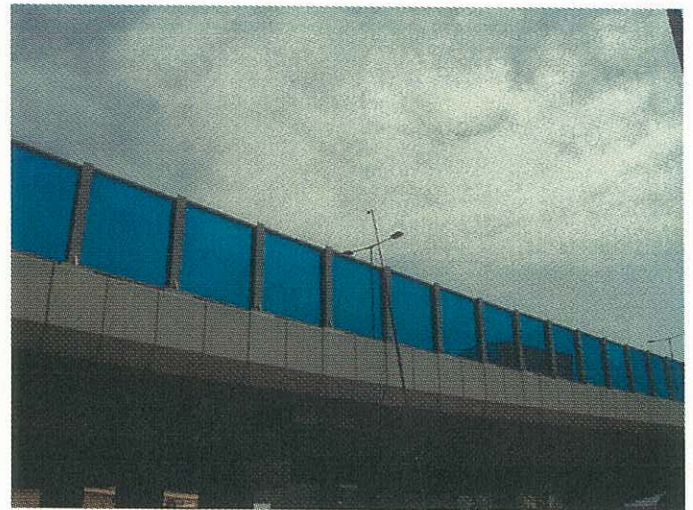
Measurement point at reference position ("after" site)
