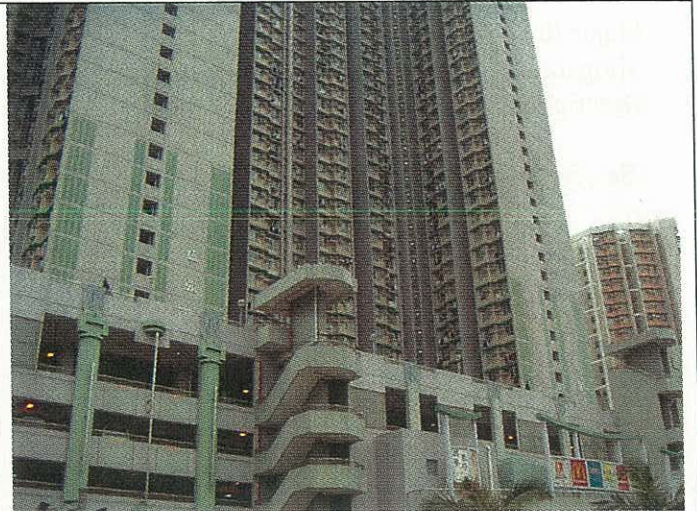
General view of the podium
