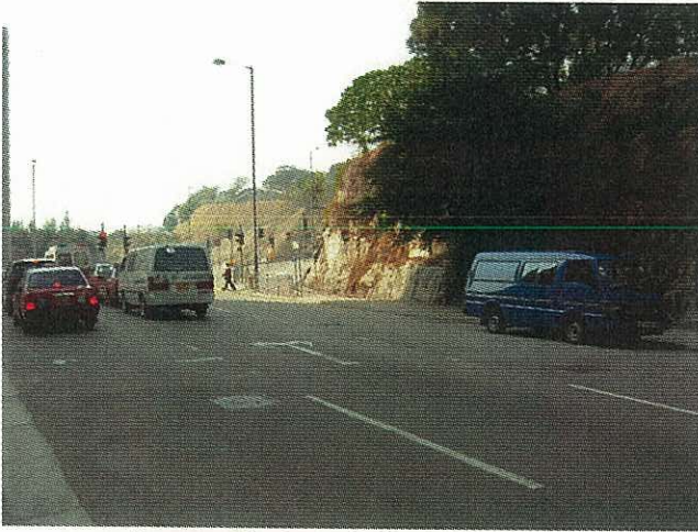
A general view of the subject road
