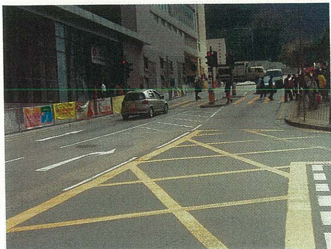
General view of the subject road
