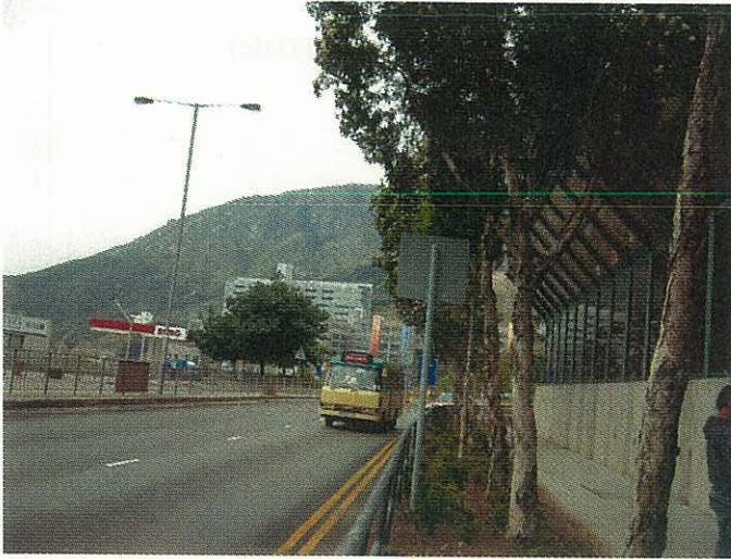
General view of the subject road
