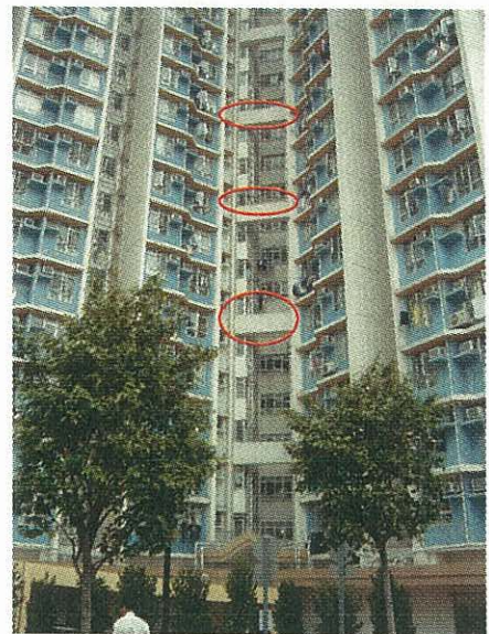
Measurement points at receiver position ("after" site)
