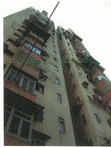
A general view of the "after" site
