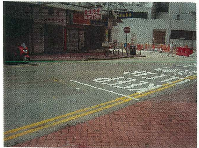
A general view of the concerned road
