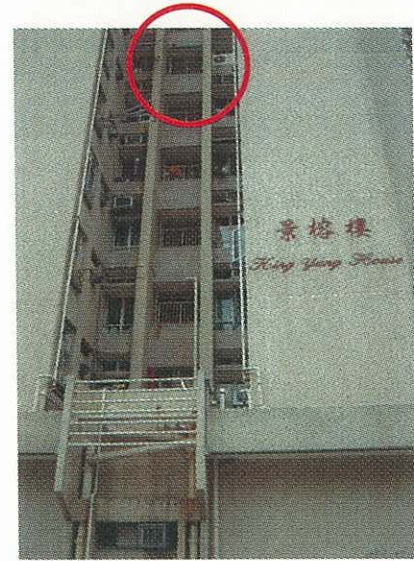
Measurement point at receiver position, low level - 6/F ("after" site)
