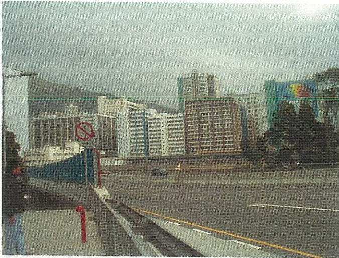
General view of the mitigation measure at "after" site
