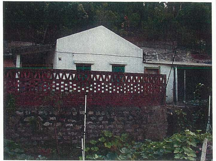
General view of the receiver site ("before" site)
