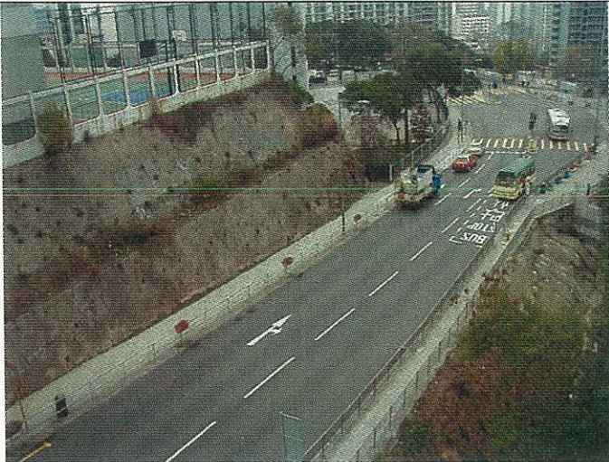
General view of the subject road
