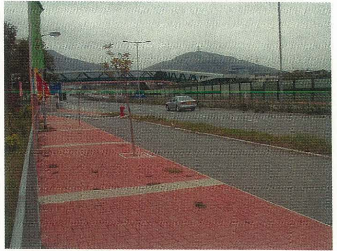
General view of the subjected road
