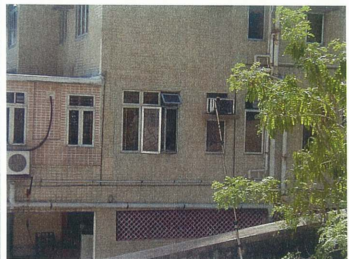
Measurement points at receiver position ("before" site)
