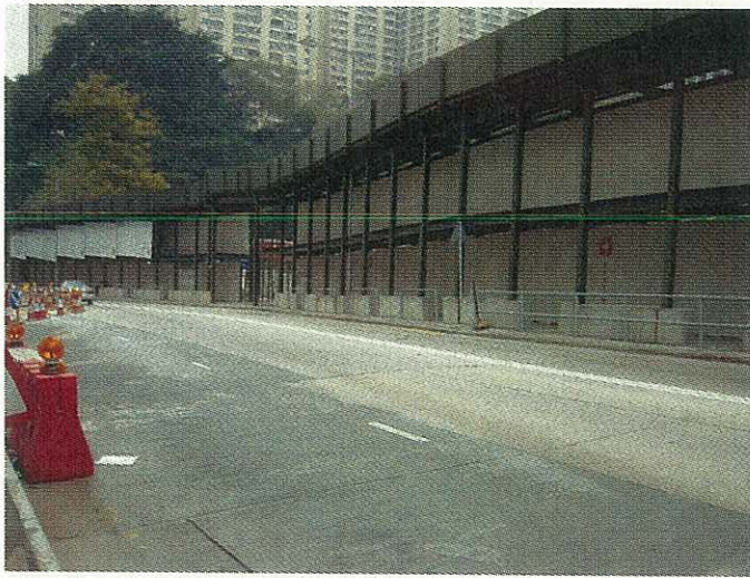
General view of the subject road
