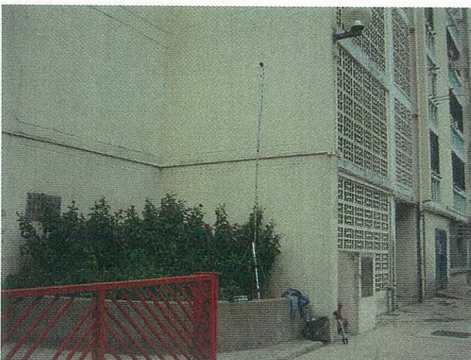
Measurement point at receiver position, low level - 1/F ("after" site)
