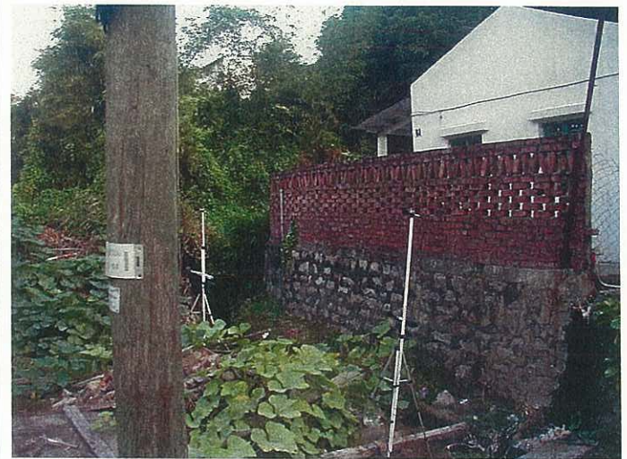
Measurement points at receiver position ("after" site)
