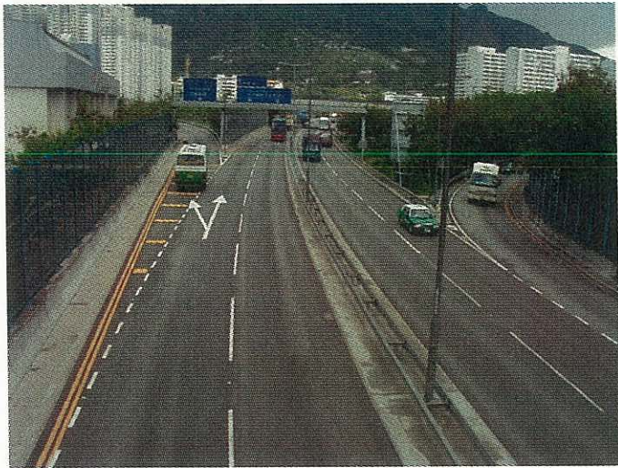
General view of the subject road
