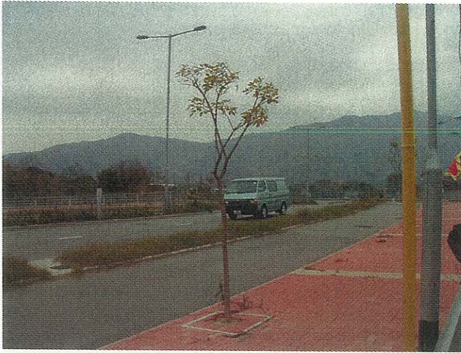
General view of the subjected road
