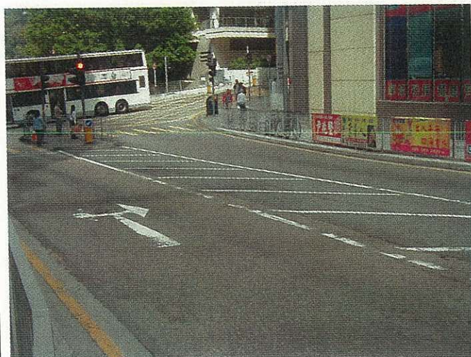
General view of the subject road
