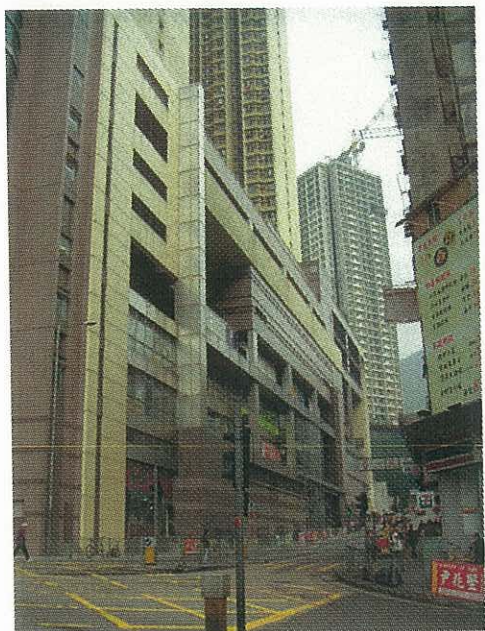
General view of the podium
