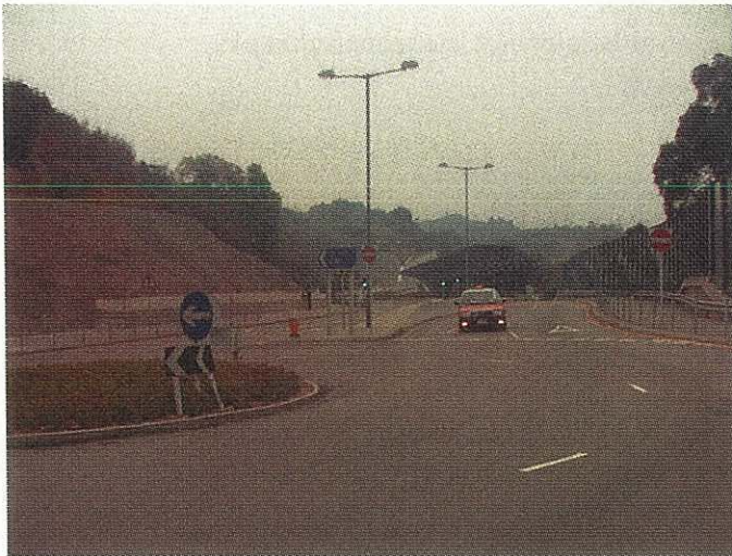
General view of the subject road
