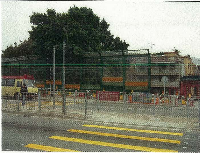
General view of the subject road and cantilever barrier
