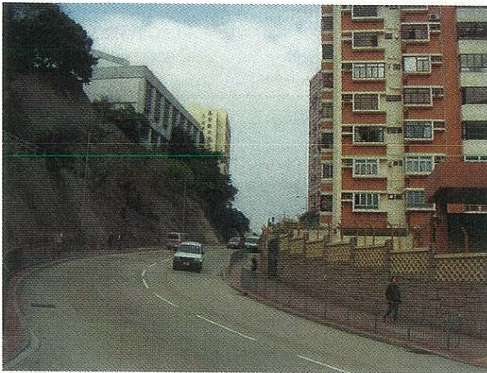
A general view of the concerned road
