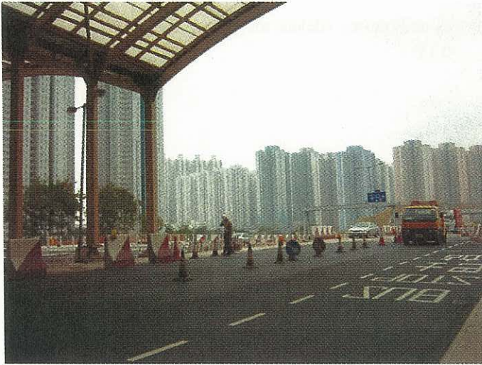
General view of the subject road
