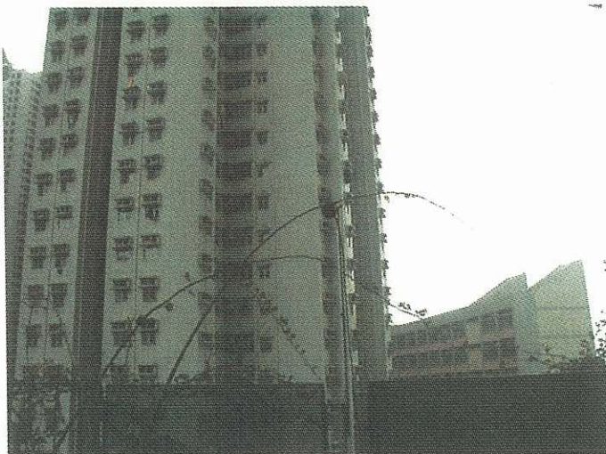
Measurement point at reference position ("after" site)
