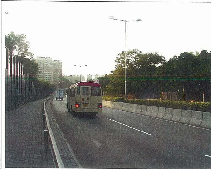
General view of the subject road
