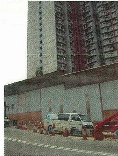
General view of the cantilever barrier
