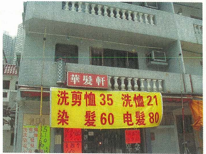
General view of the "after" site
