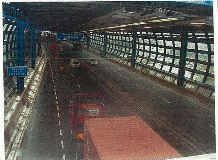
General view of the subject road
