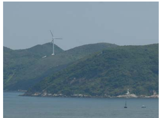
First commercial-scale wind power station, Lamma Winds , on Lamma Island.
