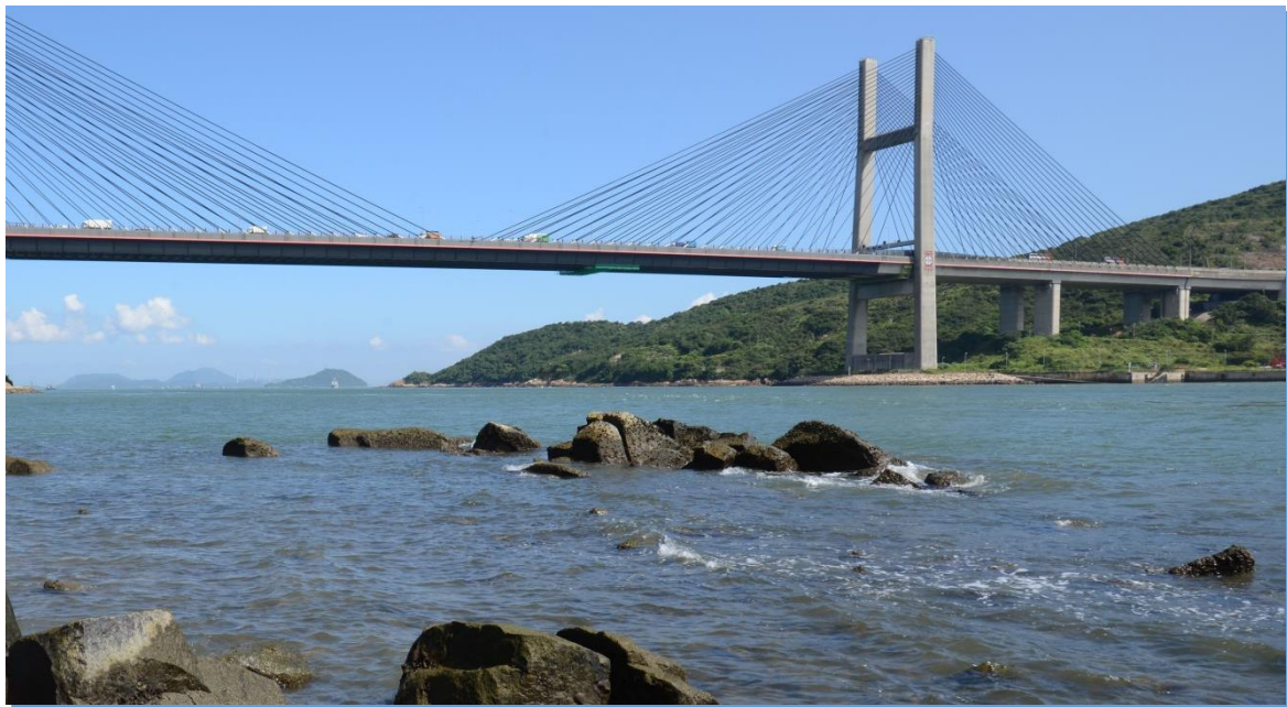
Kap Shui Mun Bridge in the Western Buffer Water Control Zone
