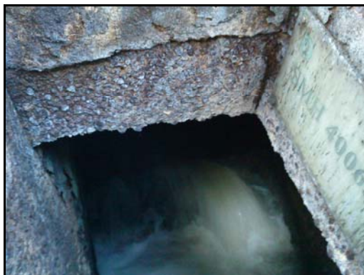
Photo 3 – Cross connection between stormwater drainage and sewerage systems (Fu Yung Street in Tsuen Wan)
