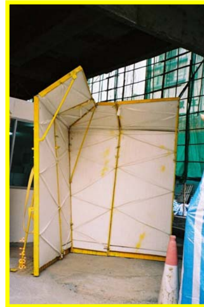
▲ Use of movable barrier to abate noise coming out from the use of noisy equipment
