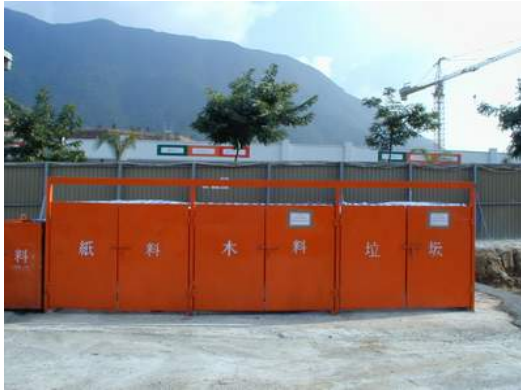
▲ Set up waste sorting and segregation area
