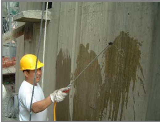
▲ Spray water before grinding
