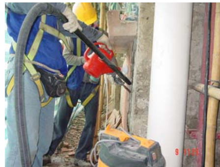
▲ Extract dust with the use of vacuum cleaner while breaking.
