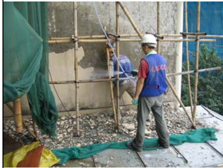
▲ Spray water while breaking
