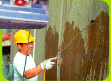
Dampen works surface
