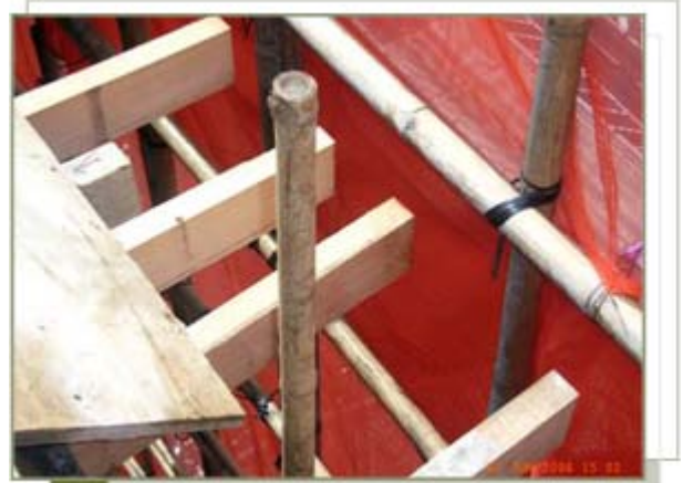
Bamboo poles are cut close to the node or their ends are wrapped up
