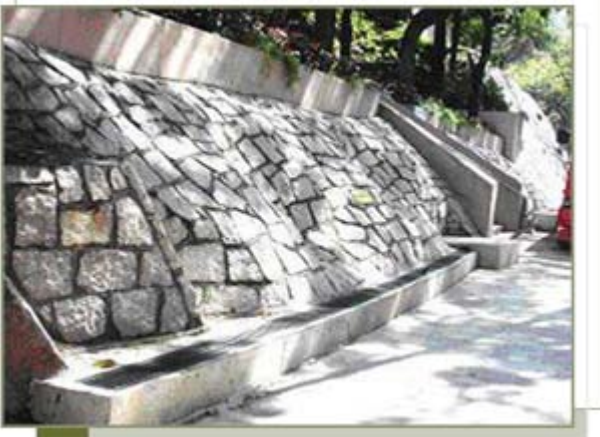
Conduct slope improvement work to enhance water runoff from slope
