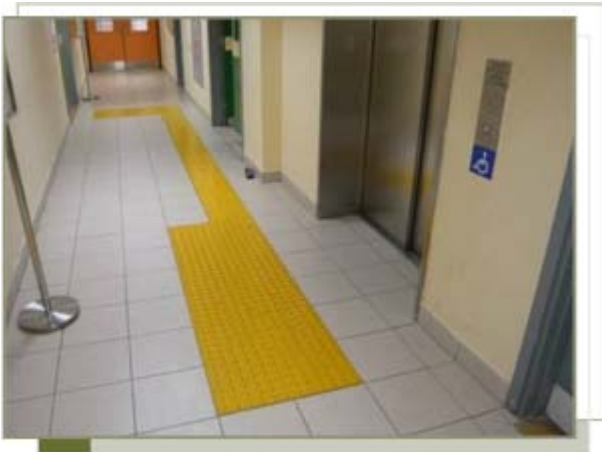
Passenger lift and tactile paths allow all building users to move easily from one floor to another
