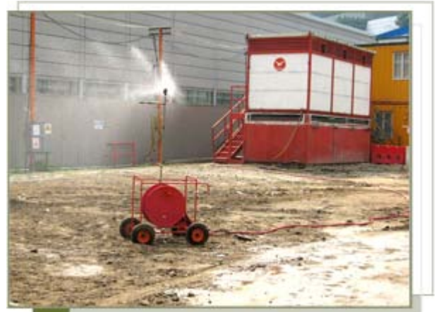
Using mobile sprinkler to minimise fugitive dust emission
