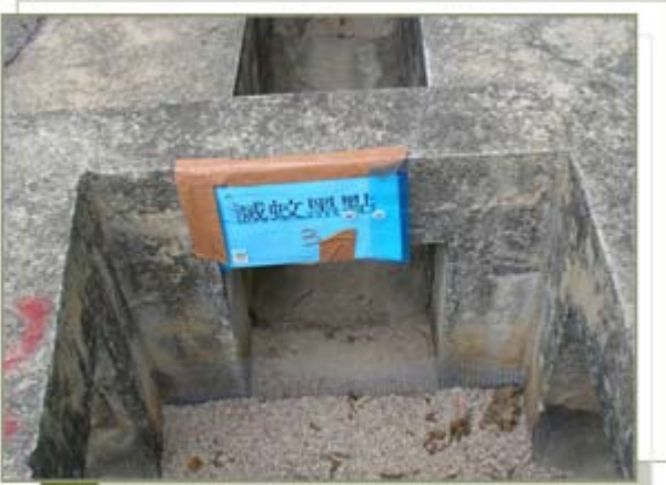
Catch Pit is filled with granular material to avoid stagnant water and so eliminates a black spot for mosquito breeding
