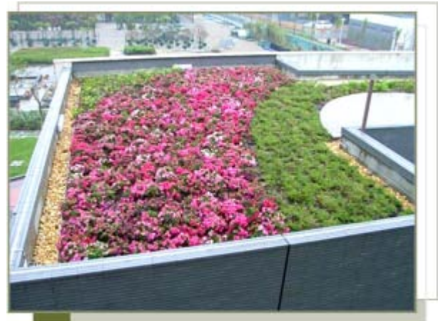
Green roof project at Tat Tung Road Garden
