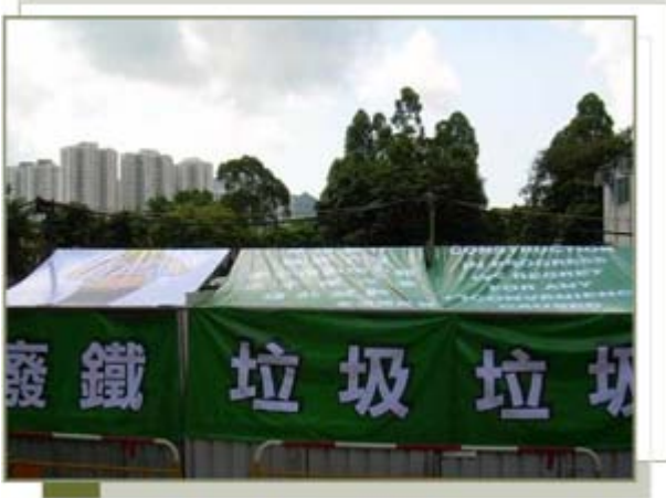
On-site Construction Waste Sorting
