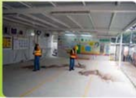
Use Floor Sweeping Compound to Minimize Water Usage 5
