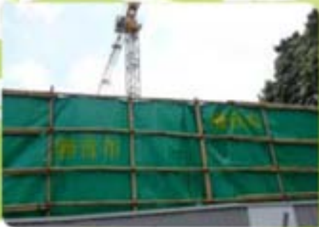
Sound Barriers around Construction Site 2
