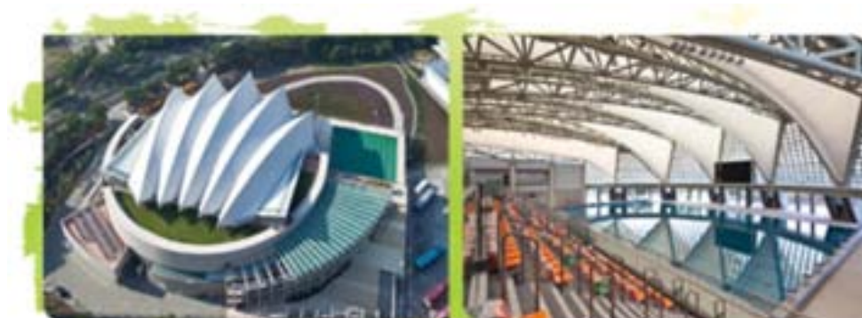
Swimming Pool Complex in Tung Chung
