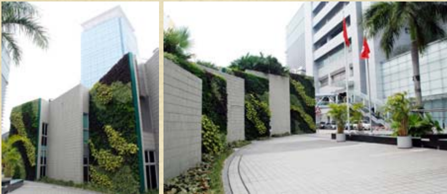
Vertical Green Walls at the EMSD Headquarters
