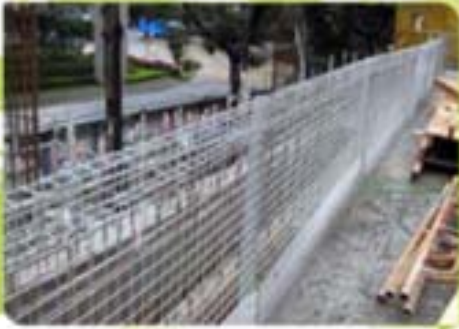
Reuse of Metal Fencing from Previous Projects 4
