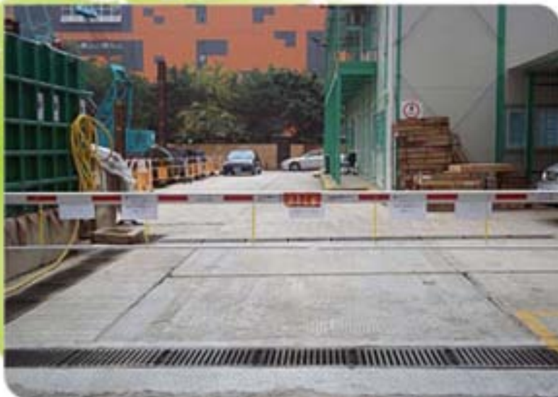
Hard-paved Construction Site
