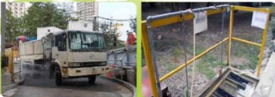
Wheel Washing at Site Exit 3
