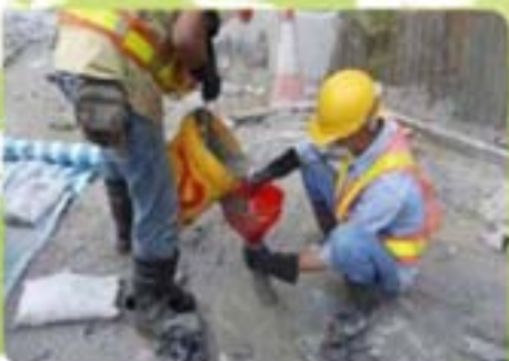
Use of Chemical Expansion Agent for Breaking Rocks 3
