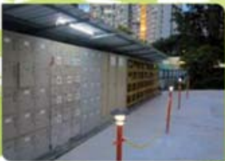
Solar LED Lamps for Access Lighting 4
