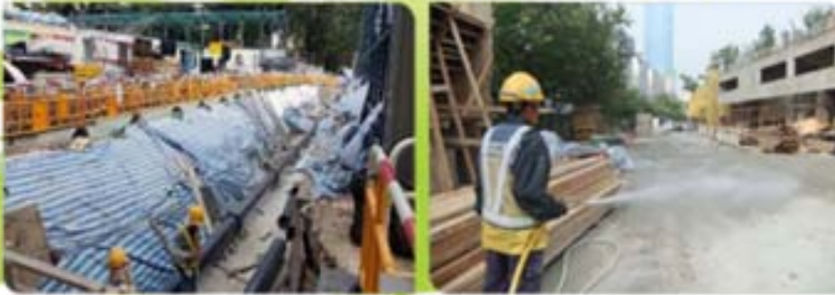
Cover on Excavated Surface 3
