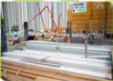
Use of Fiberglass Formwork instead of Timber Formwork 5
