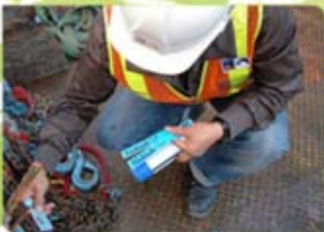
Checking Lifting Gear
