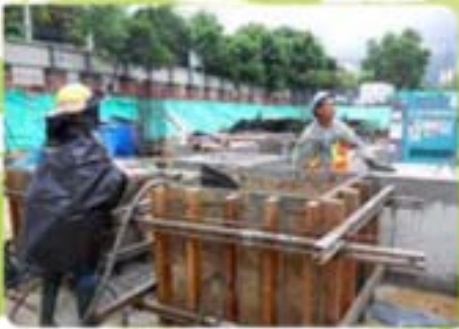
Use of Surplus Concrete for Building Block 5
