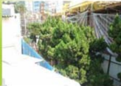
Plastic Sheets to Protect Trees from Scaffolding and Construction Works 6
