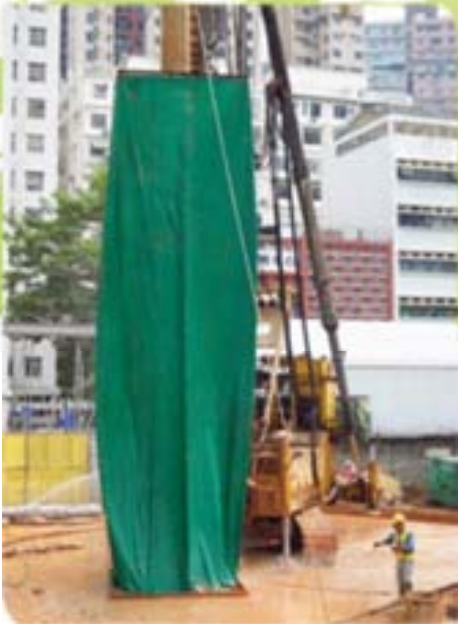
Acoustic Enclosure on Piling Plants 6
