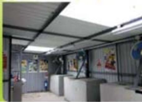
Transparent Sunroof to Make Use of Natural Light to Save Energy for Lighting 4
