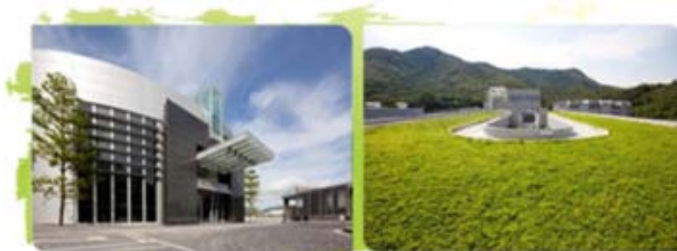
The Visitor Registration Centre of the Lo Wu Correctional Institution
