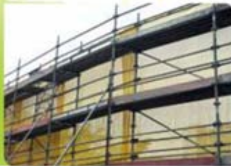
Apply Metal Scaffold instead of Bamboo Scaffold 6
