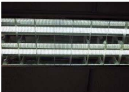
Using T10 LED light tubes
