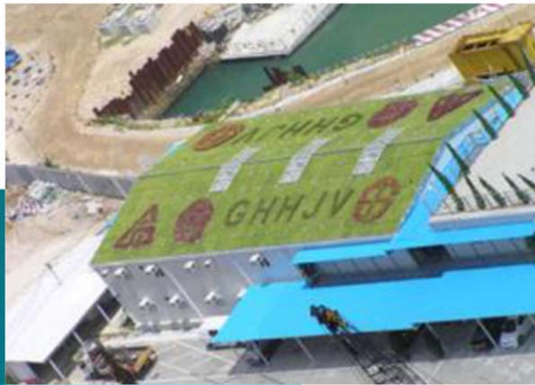
Provision of green roof at the site office
