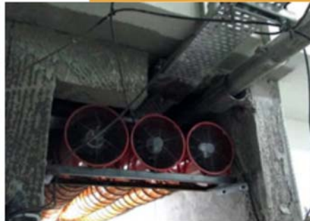
Install air blowers to improve ventilation in basement
