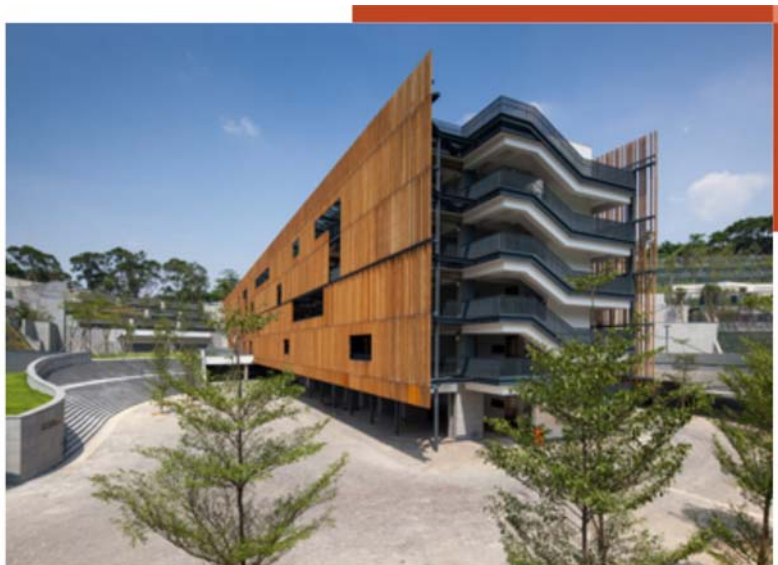
Columbarium and Garden of Remembrance at Kiu Tau Road, Wo Hop Shek
