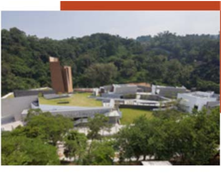
Re-provisioning of Wo Hop Shek Crematorium
