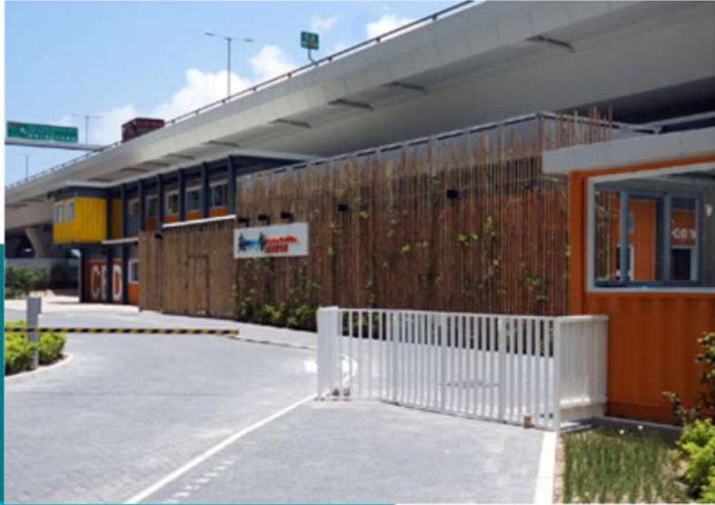
Entrance of the Energizing Kowloon East Office
