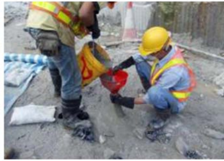
Use chemical expansion agent to break rocks
