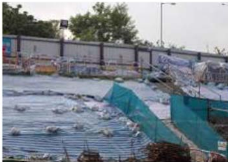
Cover exposed soil slope
