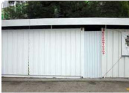
Metal roof and air gap to improve office ventilation
