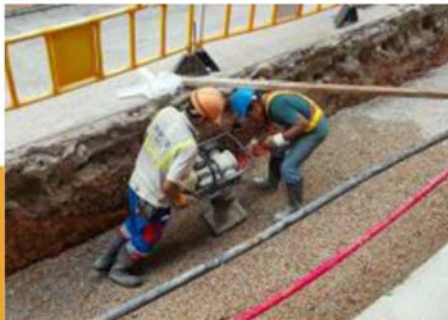
Expose earth treated by surface compaction
