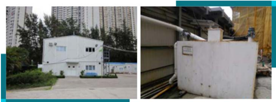
Adoption of bolt-and-nut connection at the site office to facilitate the reuse of building components
