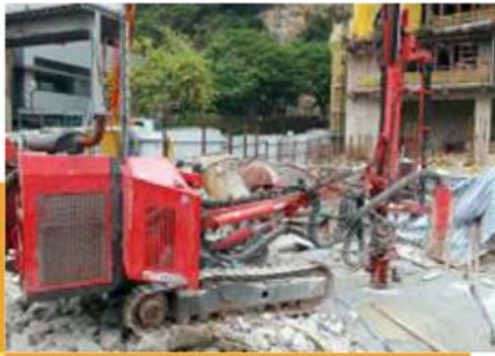
Combination of drilling machine and breakers
