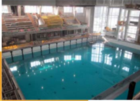
Recycling water for pool and filtration plant system test
