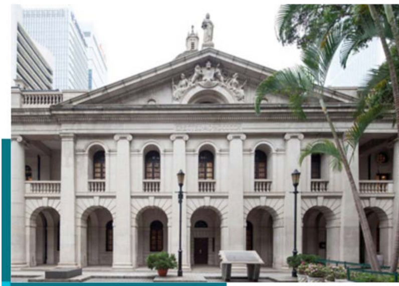
Repair and restoration Works to the exterior of the building will be carried out
