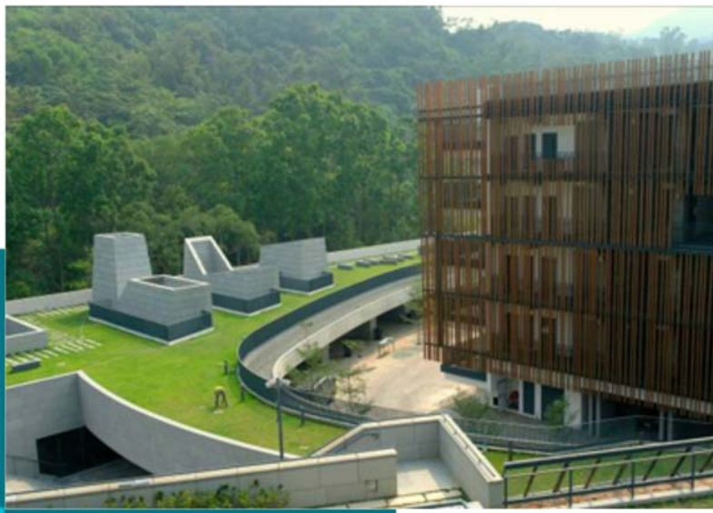
Timber screen shielding of the niches
