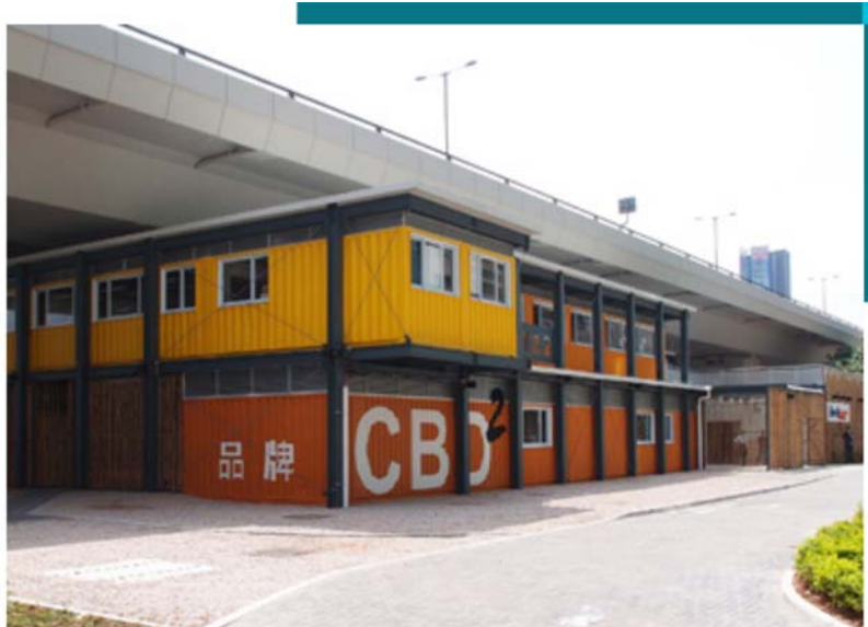
Building structure hidden under the Kwun Tong Bypass to avoid heat gain
