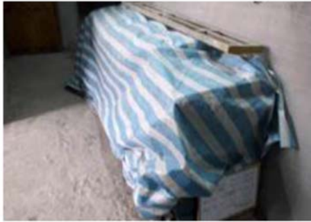
Cover over grouting station and stockpile of cement
