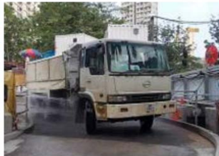
Wash Wheels at site exit
