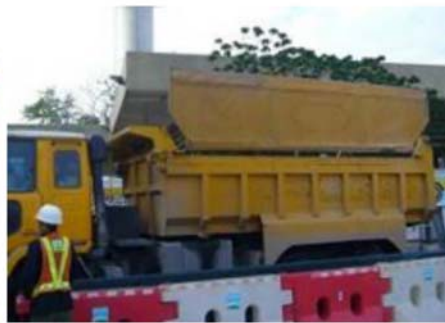
Cover dump trucks with mechanical shields
