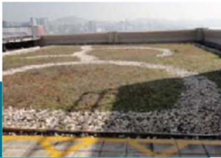
Green roof installed to reduce heat absorbed into the building
