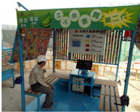
Renewable energy device with automatic thermal control for worker's resting area
