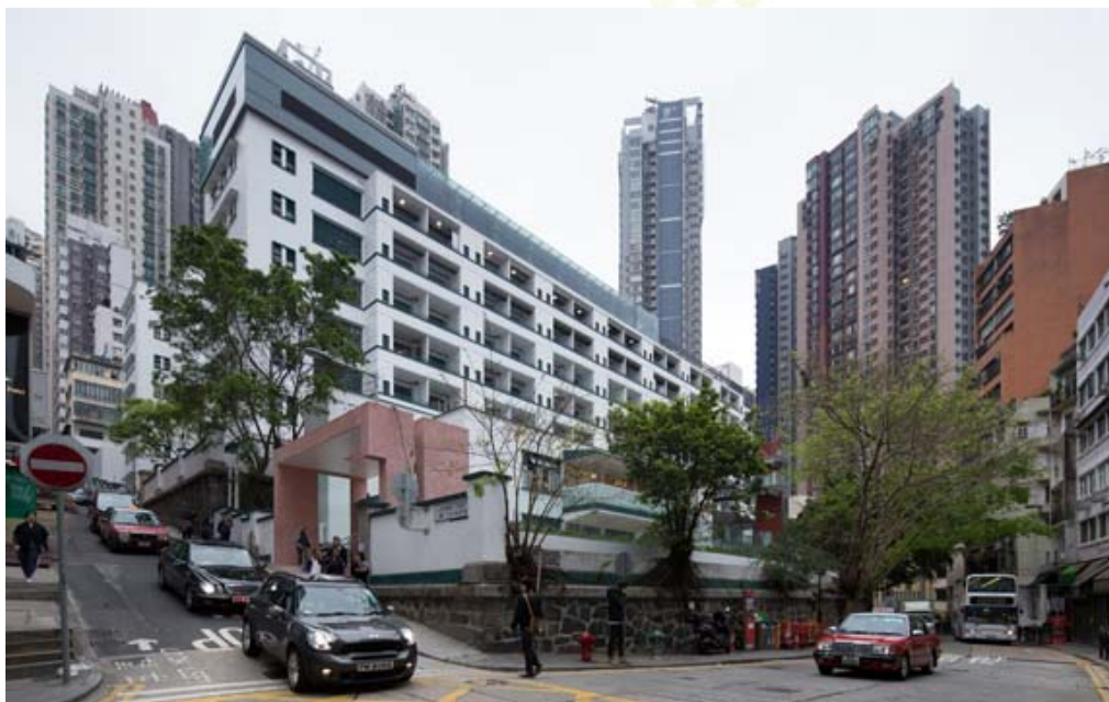
Overview of the Former Police Married Quarters
