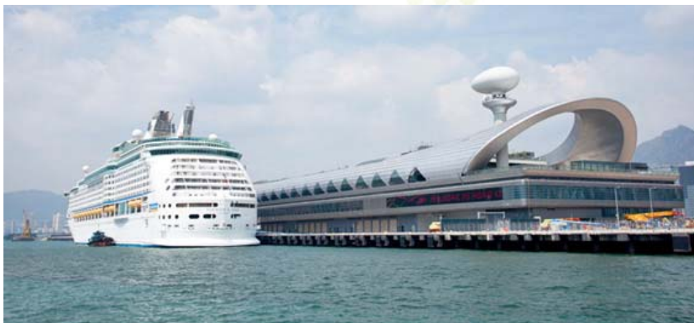
Overview of the Cruise Terminal Building
