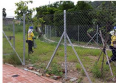
Protecting trees adjacent to site
