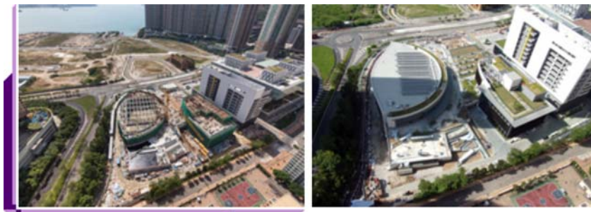
Construction of Library, Sports Center and District Open Space at Area 74 Tseung Kwan O (left: under construction, right: project completion)
