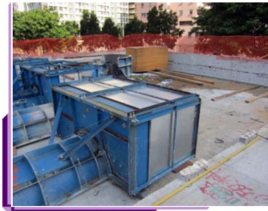
Tailor made acoustic panel for screening the noisy column concreting process
