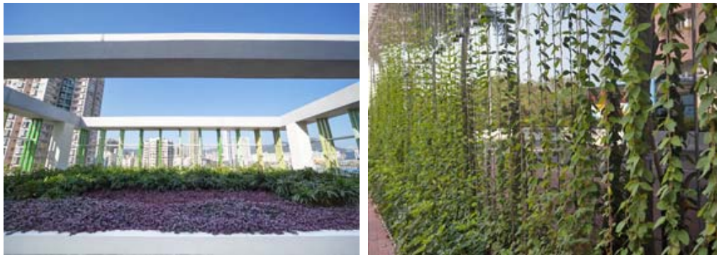
The complex has established green roofs and terraces, and vertical greening on external walls for environmental and amenity benefits
