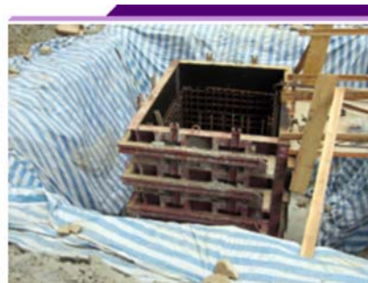
Make use of reusable steel moulds to replace timber formwork
