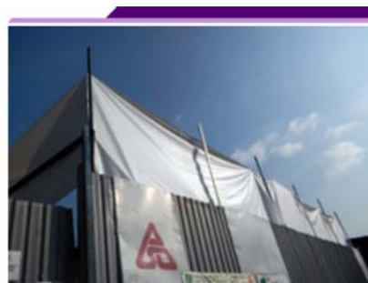
Erection of Dust Screen
