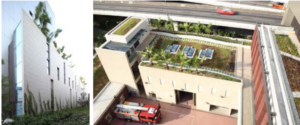
Up to 43% of green coverage has been achieved through green wall and green roofs
