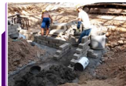
Using brick work as formwork to minimise timber usage
