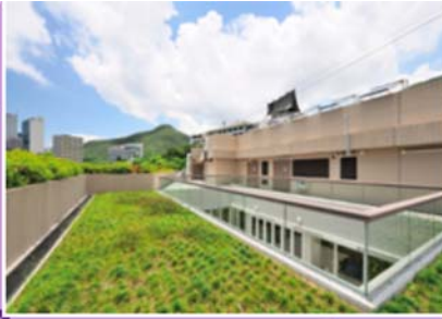
Green roof installation
