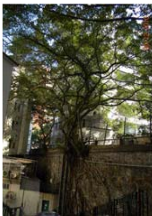
Preservation of existing retaining walls together with the unique wall trees
