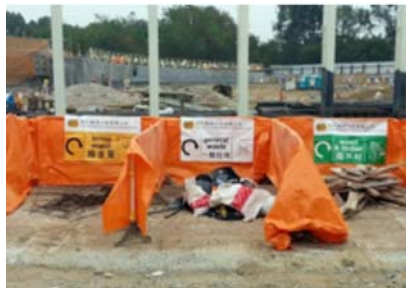
Designated area for on-site waste sorting
