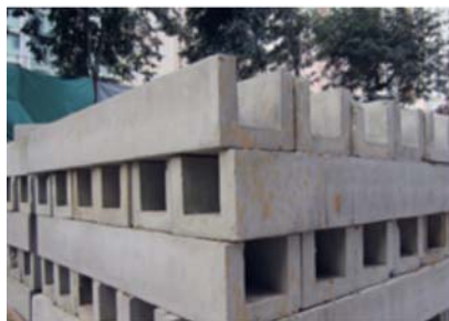
Adopting Pre-cast U-channel to minimise in-situ formwork and concreting work
