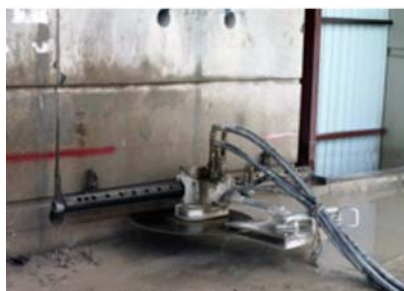
Demolition using low-dust-impact saw-cutting method
