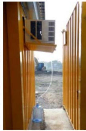
Collect water from air conditioner for reuse
