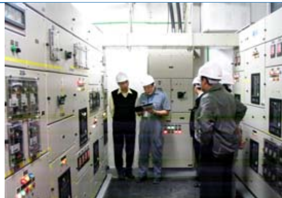
Electrical Safety Inspection
