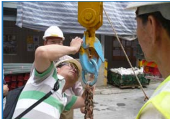
Site safety inspection for lifting operations
