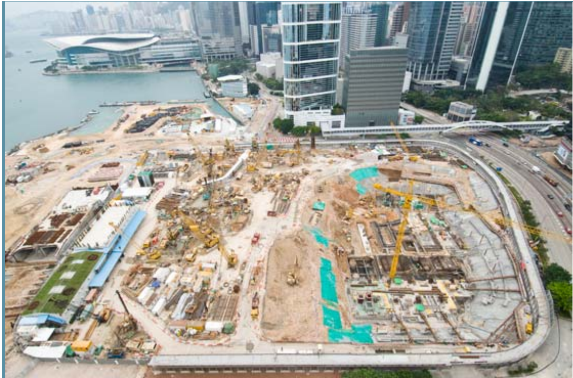
Tamar Development Project under construction
