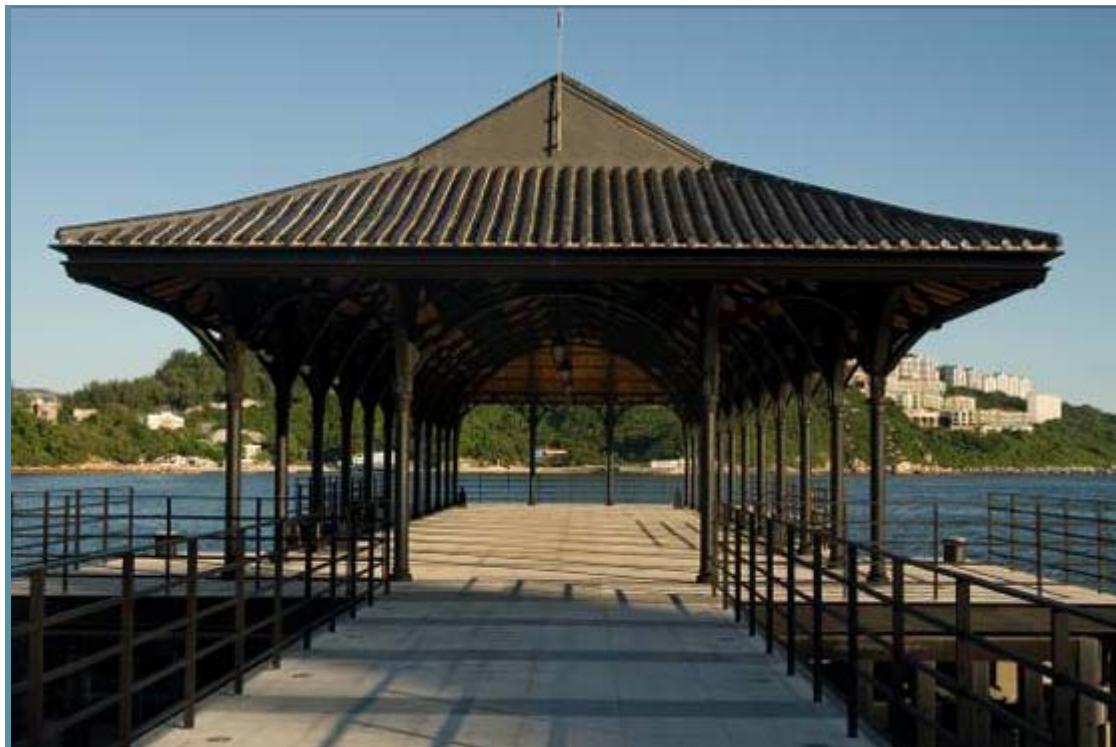
The new Blake Pier at Stanley Waterfront Promenade
