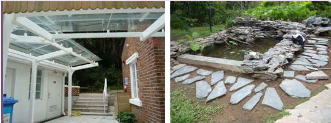
After renovation - Lung Fu Shan Environmental Education Centre
