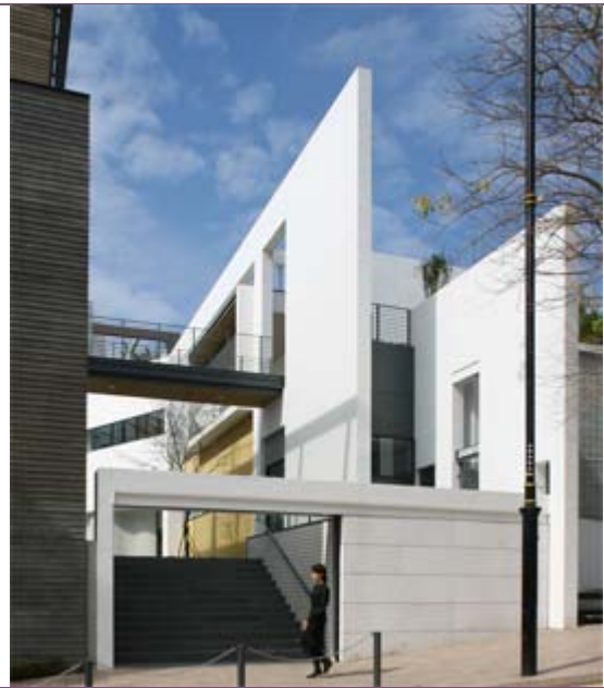
Grand Award (New Construction Category) - Stanley Municipal Services Building (Stanley Complex)
