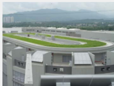
Green Roof of Dormitory Block
