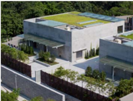
Green roofs on the service halls
