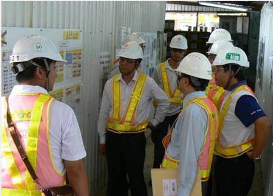
Site safety promotion by contractors
