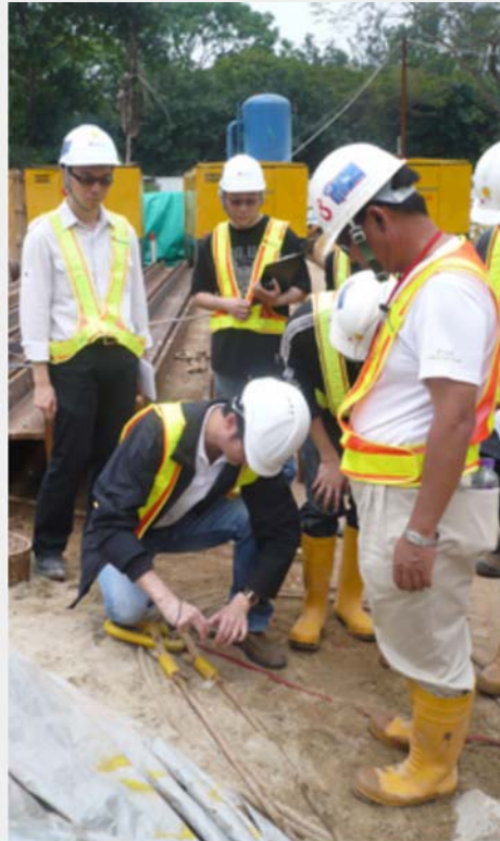
Checking the integrity of wire slings
