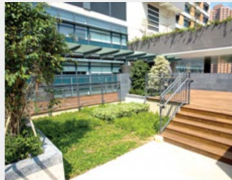
Rehabilitation Block at Tuen Mun Hospital Phase II
