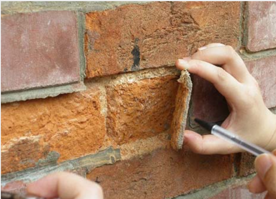
Fair Face Red Brick Façade
