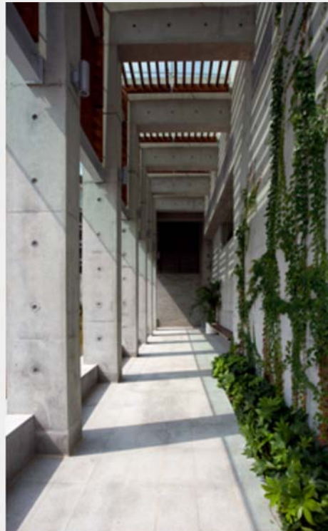
Vertical greening on the building
