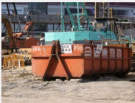
Onsite waste sorting
