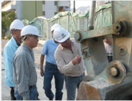
Site safety inspection for mechanical plant
