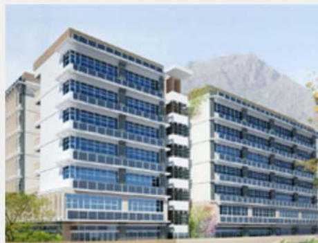
View of the school premises from South-Western direction
