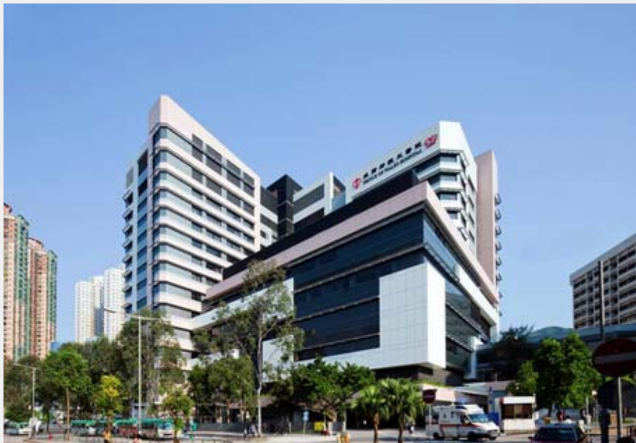
Prince of Wales Hospital Extension Block
