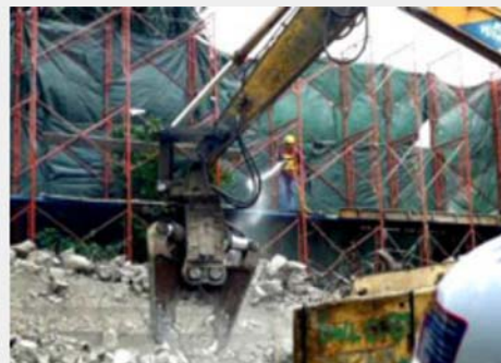
Use of hydraulic crusher
