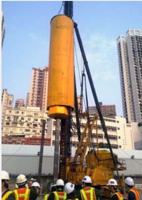
Acoustic enclosures on piling plants
