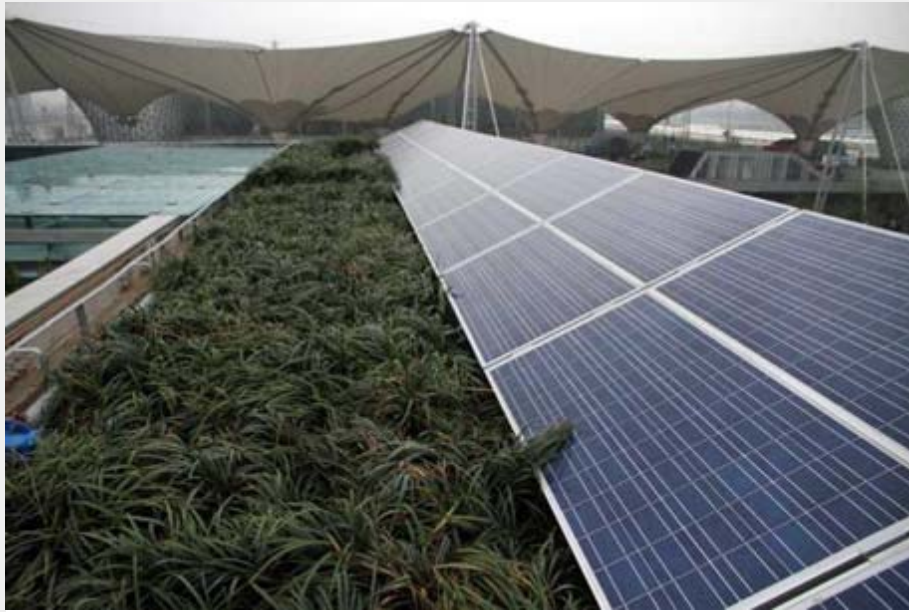
Solar Panel on roof with roof greening
