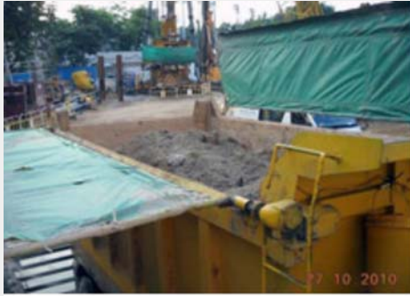
Use of mechanical cover for trucks
