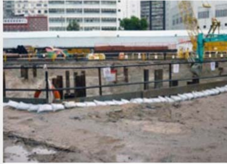
Excavated materials reused for making sandbags and backfilling
