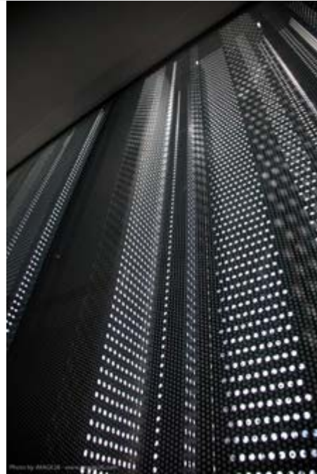
Perforated Panel to allow natural lights entering the interior of the HK Pavilion
