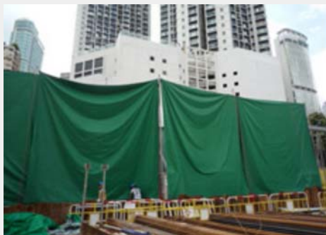
Acoustic mat for noisy work
