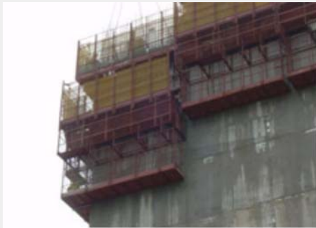
Use of system formwork
