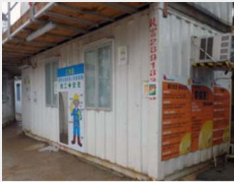
White reflective paint to lower room temperature
