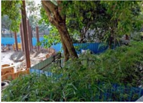
Hoardings erected for tree protection zones
