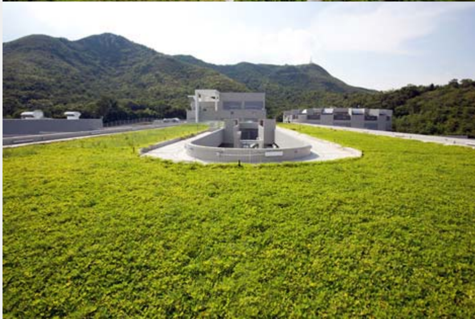
Redevelopment of Lo Wu Correctional Institution - Green Building Award 2010 - Grand Award(New Buildings Category - Hong Kong Institutional / Community Project)
