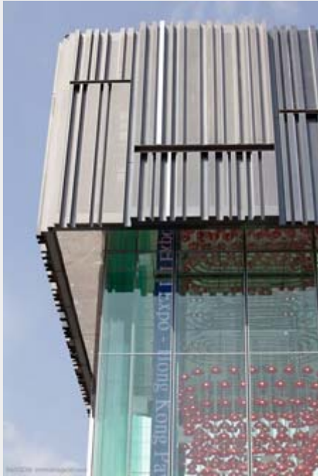
Perforated Panel to allow natural lights entering the interior of the HK Pavilion
