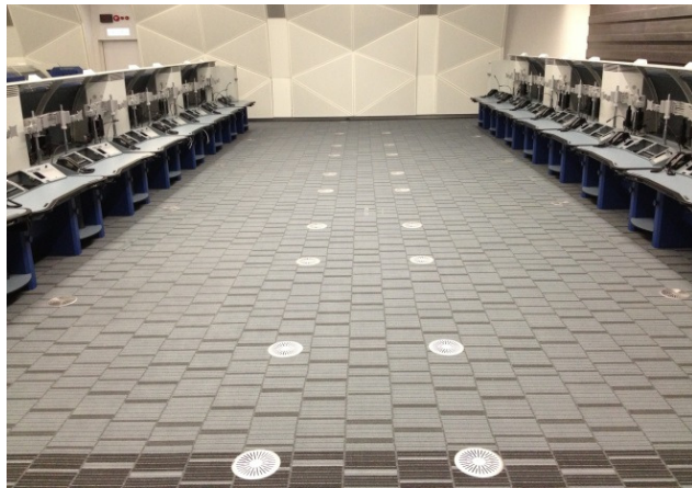
Figure 5-6: Separation of air-conditioning for equipment and occupant
