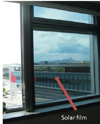
Figure 5-12: Solar films are installed in strategic locations to reduce sunlight and heat
