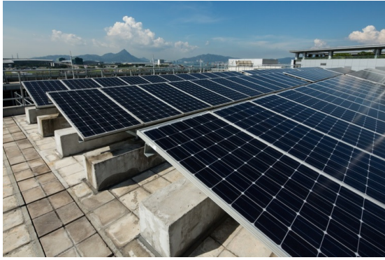
Figure 5-3: Approximate 130 m 2 of Photovoltaic Panels
