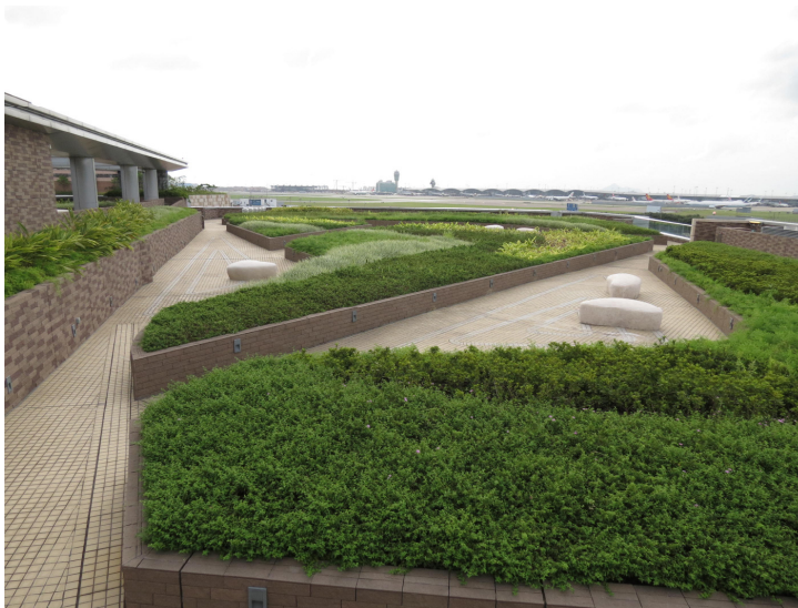
Figure 5-4: Green roof of CAD Headquarters
