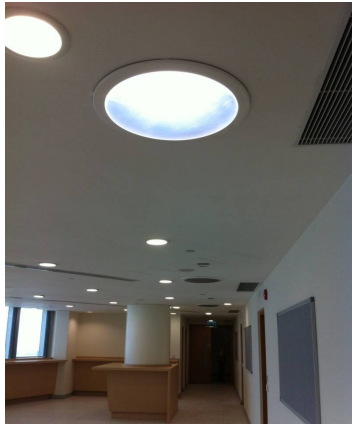
Figure 5-1: Light pipes at the roof of ATC Building (viewing from underneath)
