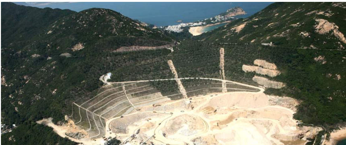
Shek O Quarry rehabilitation work in progress
