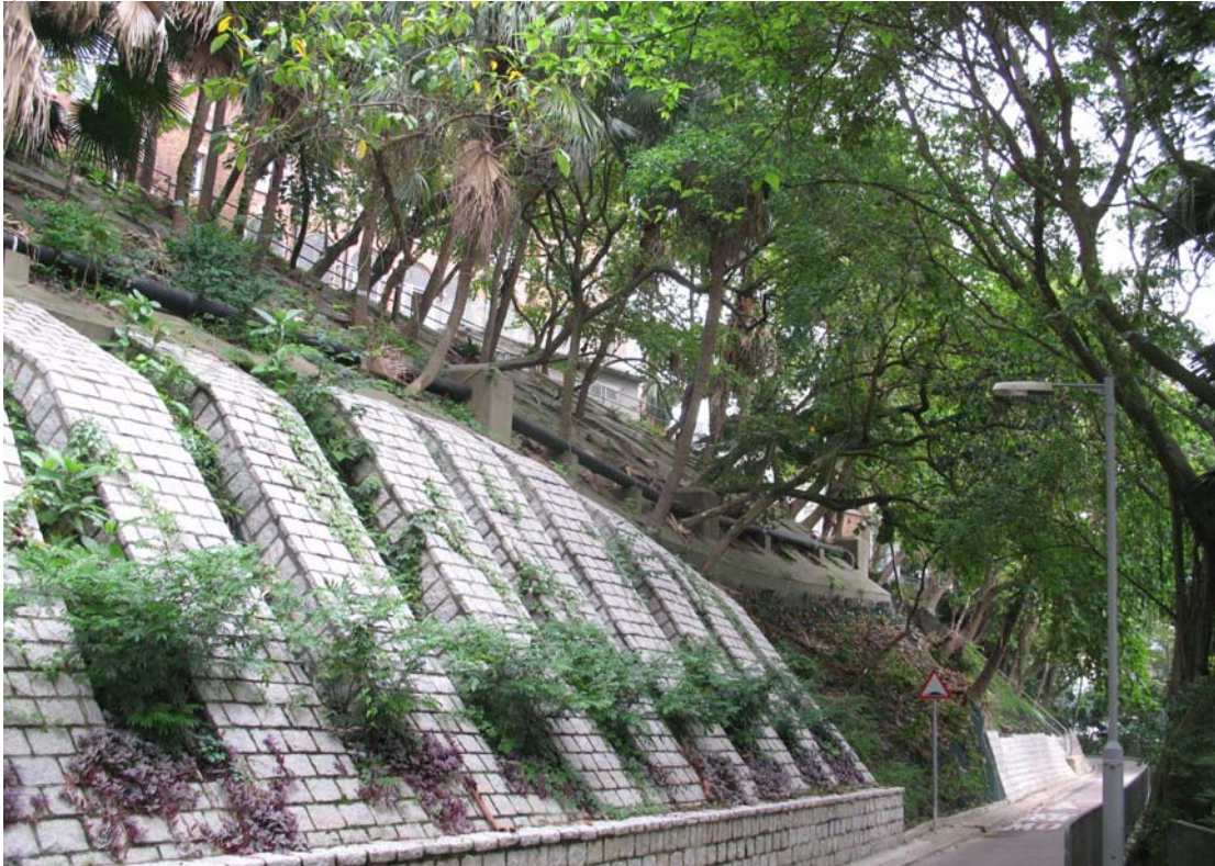
Landscaping work on an LPM slope along Bowen Road shows tree preservation, hard landscaping and at the same time maximizing planting opportunity.
