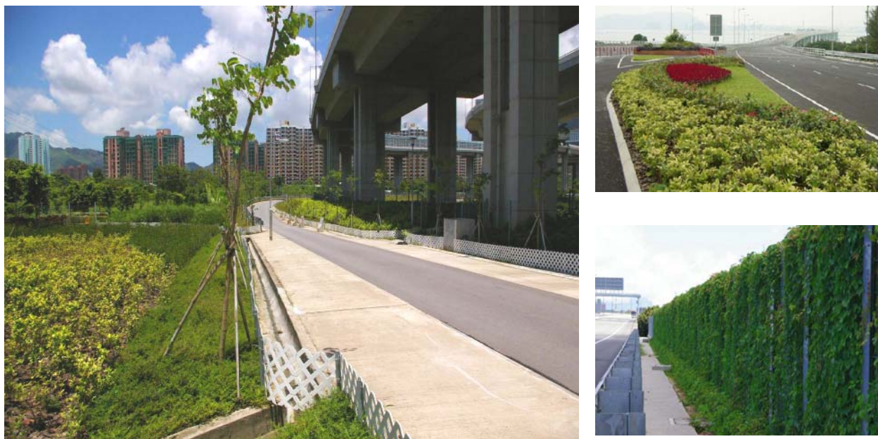
Greening Works for Deep Bay Link
