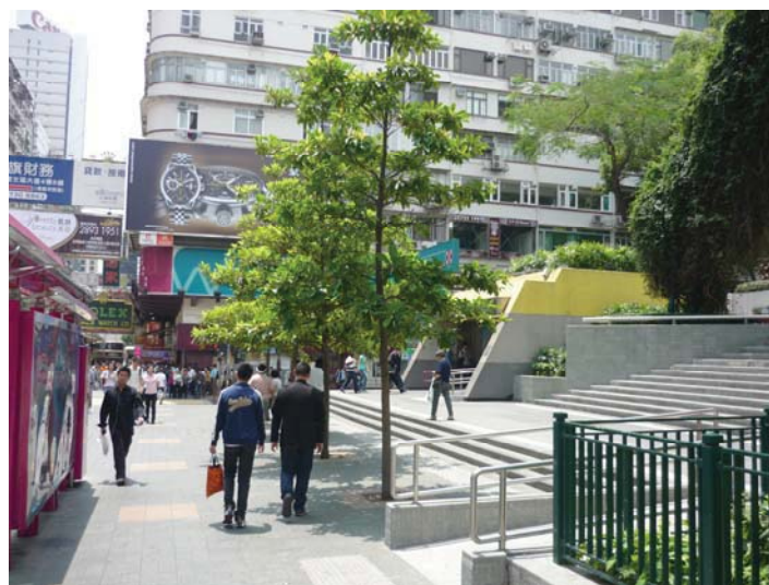
Improvement Works near Tsim Sha Tsui MTR Station
