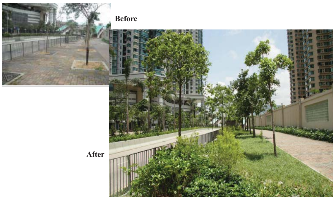
Greening works under the GMP for Mong Kok and Yau Ma Tei – Hoi Fai Road
