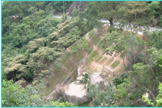
As-built photo taken in August 2003, concrete grill structure can be seen from distance.
