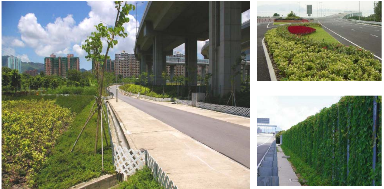
Greening Works for Deep Bay Link
