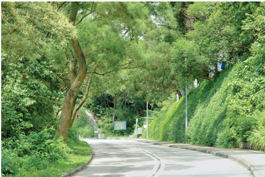
Greening work on the LPM slopes along South Lantau Road, Lantau
