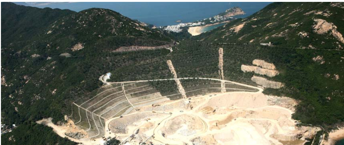
Shek O Quarry rehabilitation work in progress
