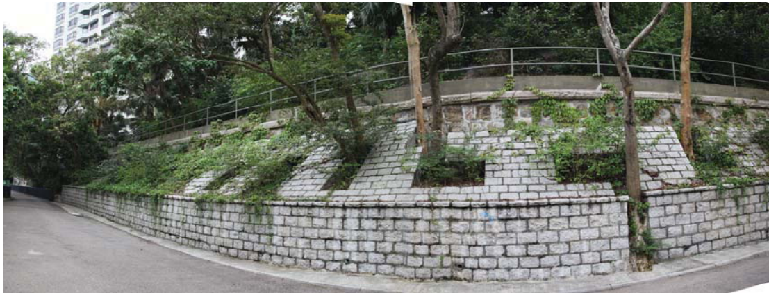
Hard landscaping work along Bowen Road blends with the environment
