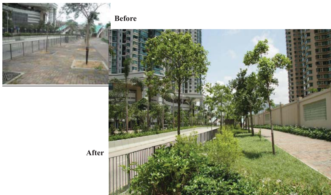
Greening works under the GMP for Mong Kok and Yau Ma Tei – Hoi Fai Road
