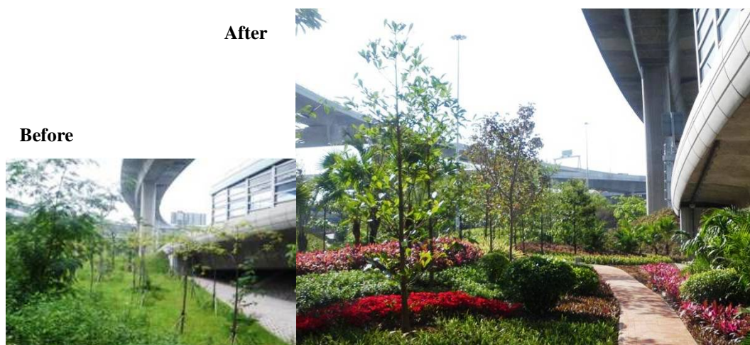
Greening works under the GMP for Sham Shui Po – Lai Po Road
