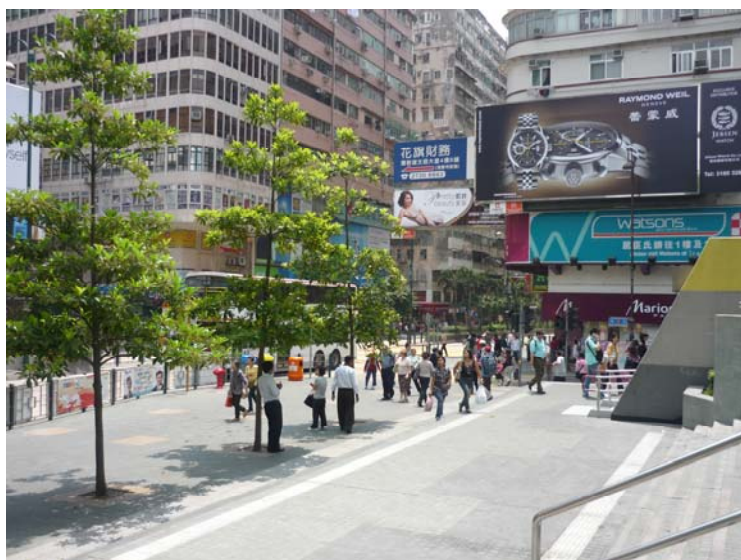
Improvement Works near Tsim Sha Tsui MTR Station
