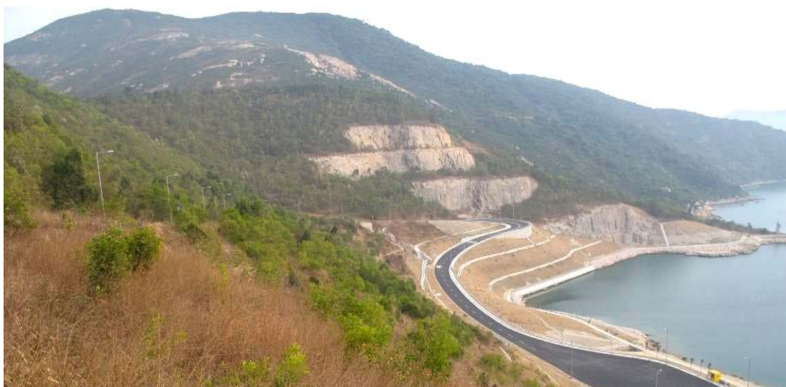
A view of Shek O Quarry
