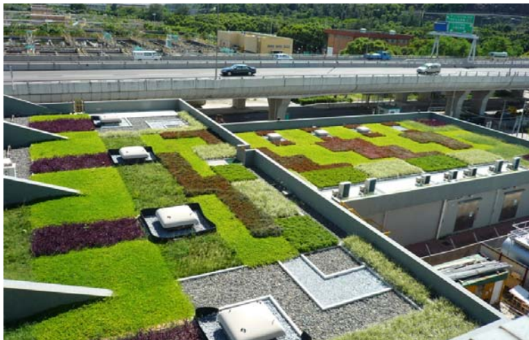
Roof greening at Shatin Sewage Treatment Works
