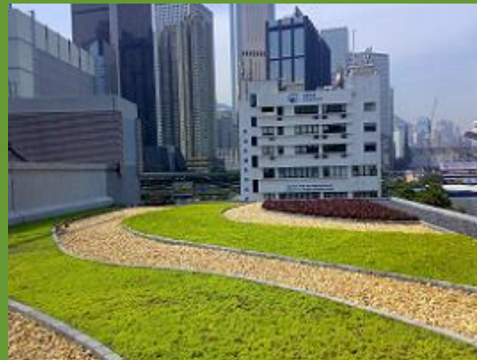
Green roof of the Wan Chai East Sewage Screening Plant
