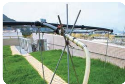
Run-off mitigation study of green roof
