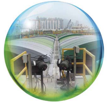
昂船洲污水處理廠－已覆蓋的沉澱池 SCISTW - sedimentation tanks with covers
