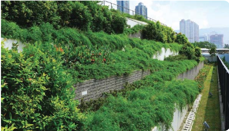
九龍城二號污水泵房的垂直綠化 Vertical greening at Kowloon City SPS No. 2
