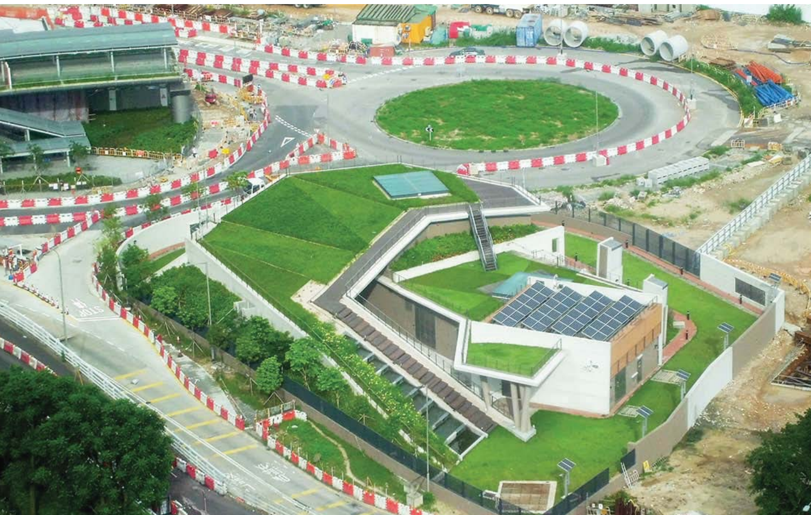
九龍城一號污水泵房鳥瞰圖 Bird's-eye view of Kowloon City SPS No. 1
