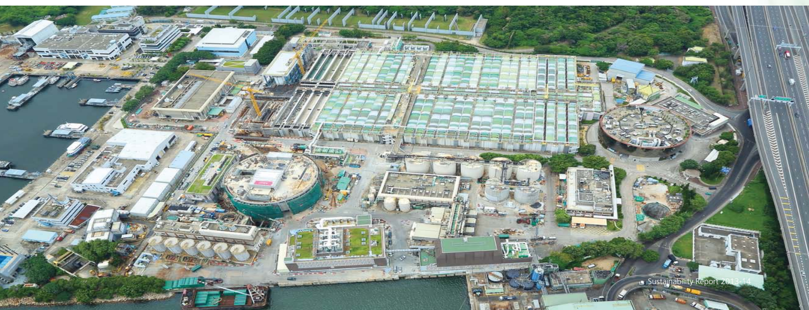
昂船洲污水處理廠－已覆蓋的沉澱池 SCISTW - sedimentation tanks with covers
