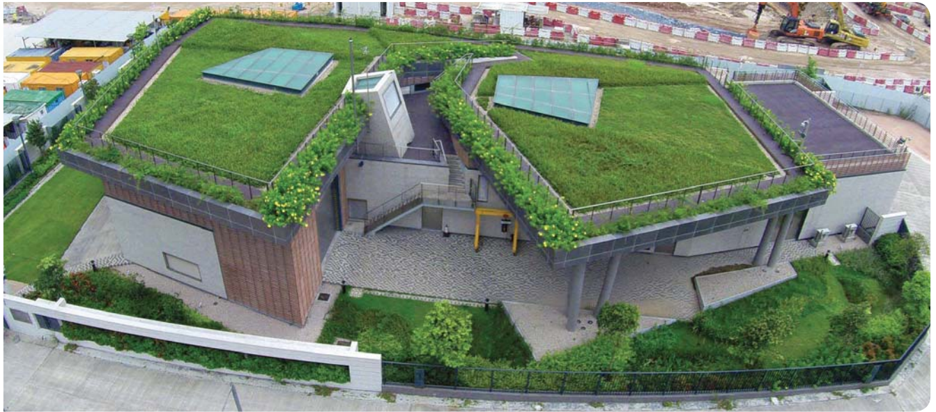
九龍城二號污水泵房鳥瞰圖 Bird's-eye view of Kowloon City SPS No. 2
