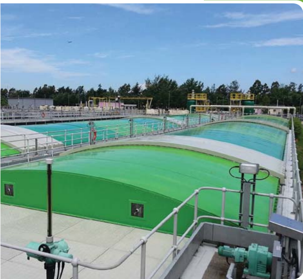
初級沉澱池的密封玻璃纖維強化塑膠蓋 Fiberglass reinforced plastic covers for primary sedimentation tanks
