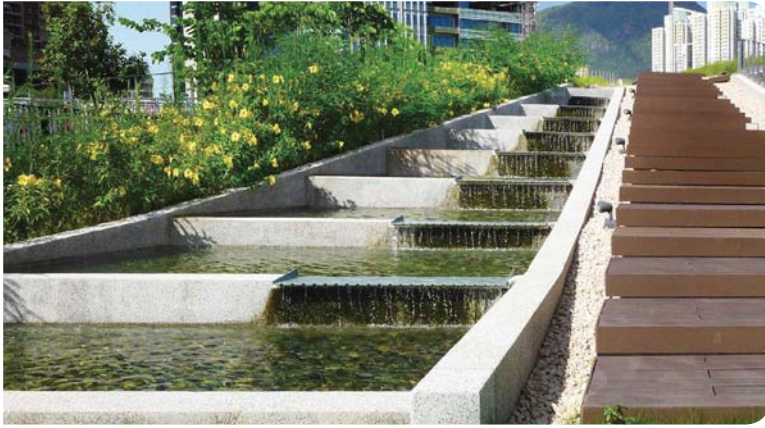
九龍城一號污水泵房的水景 Water feature at Kowloon City SPS No. 1
