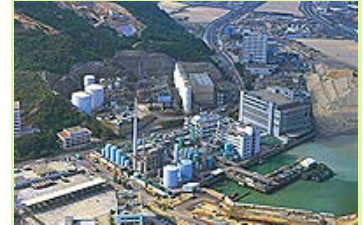
Chemical Waste Treatment Centre, Tsing Yi
