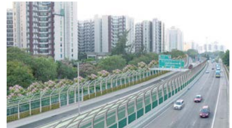
Noise Barriers erected at busy roads to protect nearby dwellings from traffic noise.
