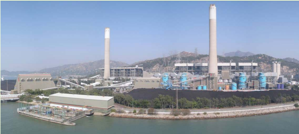
The coal-fired generation units of Castle Peak Power Station B has retrofitted with emission reduction facilities (The four flue gas desulphurisation plants are in blue at the front.) – Courtesy of CLP Power Hong Kong Limited.
