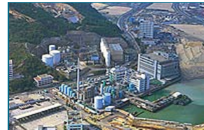
Chemical Waste Treatment Centre, Tsing Yi
