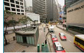
Roadside Air Monitoring Station at Central
