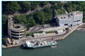
Island West Transfer Station
