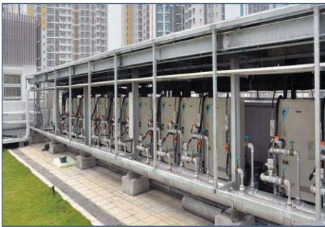
Water cooled VRV system
