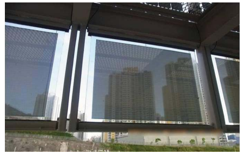
Semi-transparent amorphous PV panels
