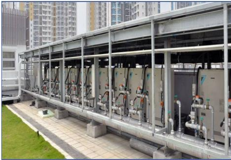
Water cooled VRV system
