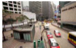
Roadside Air Monitoring Station at Central
