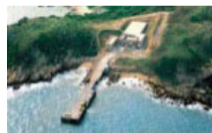
Low-level Radioactive Waste Storage Facility, Siu A Chau
