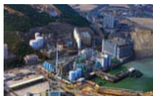
Chemical Waste Treatment Centre, Tsing Yi
