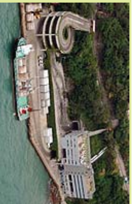
Island West Refuse Transfer Station
