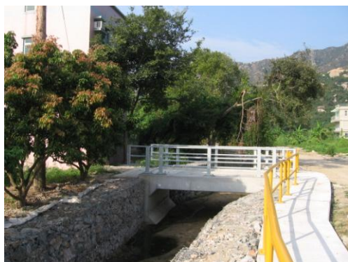
Use of natural stones for the construction of gabion wall as embankment adjacent to a stream at Lung Kwu Tan, Tuen Mun
