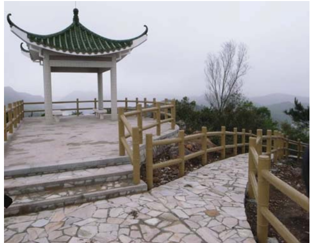
Use of natural stones for paving a walking trail leading from Sam Shing Kung to Ko Tei Teng, Kat O, Sha Tau Kok North District
