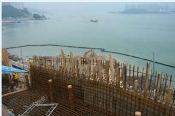
Silt curtain as water pollution nuisance abatement
