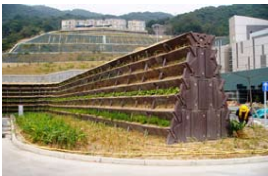
Route 8 engineered earth mound
