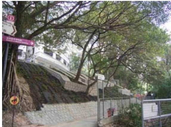
Slope No. 11SW-A/FR135 at Caine Lane – Preservation of existing trees in-situ as part of the slope upgrading works
