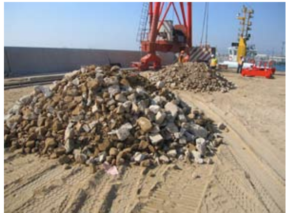
Using of recycled grade 200 rock fill from Public Filling Area as temporary road sub-base
