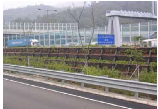
Earth mound along Yuen Long Highway north bound to Kong Sham Western Highway north bound
