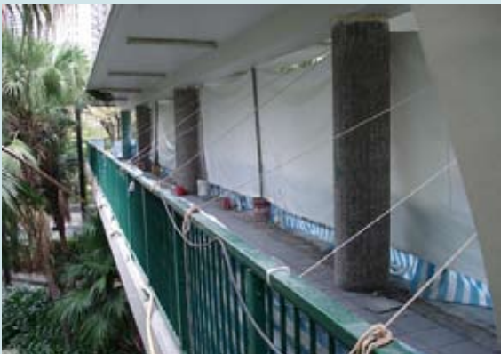
Plastic and tarpaulin sheets as dust pollution nuisance abatement
