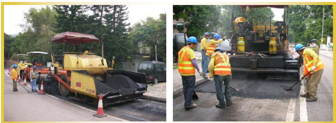
Laying of reclaimed asphalt pavement in Sai Kung
