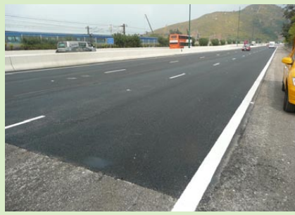
North Lantau Expressway with wearing course incorporating RAP laid under conventional polymer modified friction course
