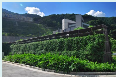
Route 8 engineered earth mound
