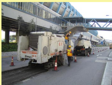
Milling of deteriorated pavement
