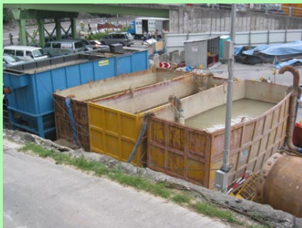
Sedimentation tanks
