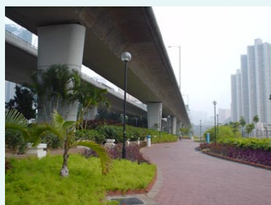
Flyover above Tsuen Wan Park
