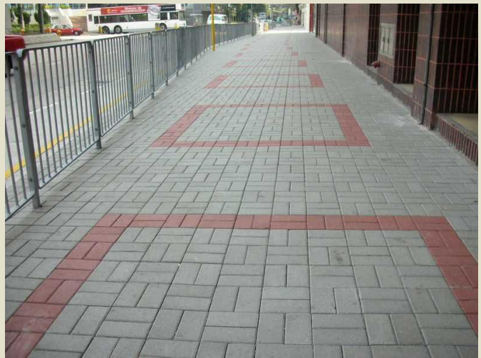
Paving blocks with glass at Wang Kwong Road
