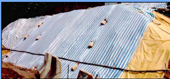
Providing cover for open stockpile
