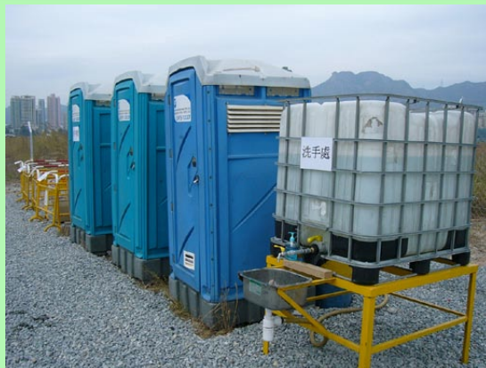
Keeping site tidy by providing sanitary facilities
