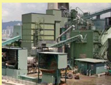
Mixing of RAP material with virgin asphalt pavement in plant
