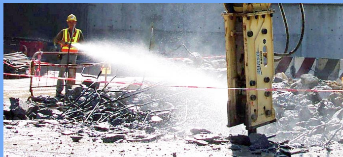
Water spraying for dust suppression
