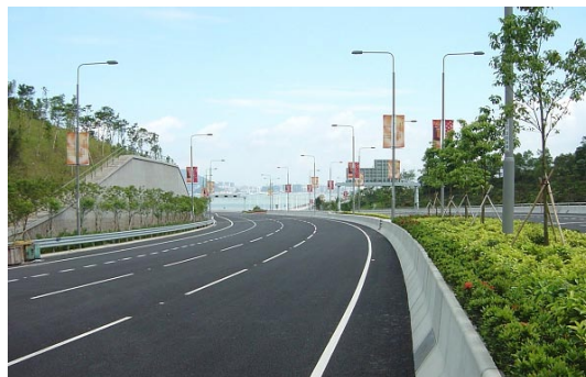
Planting to green transport corridor
