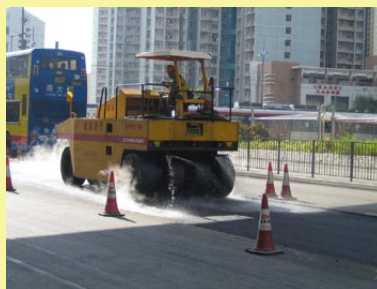
Final rubber rolling of asphalt pavement with RAP material
