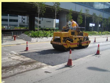
Steel rolling of asphalt pavement with RAP material
