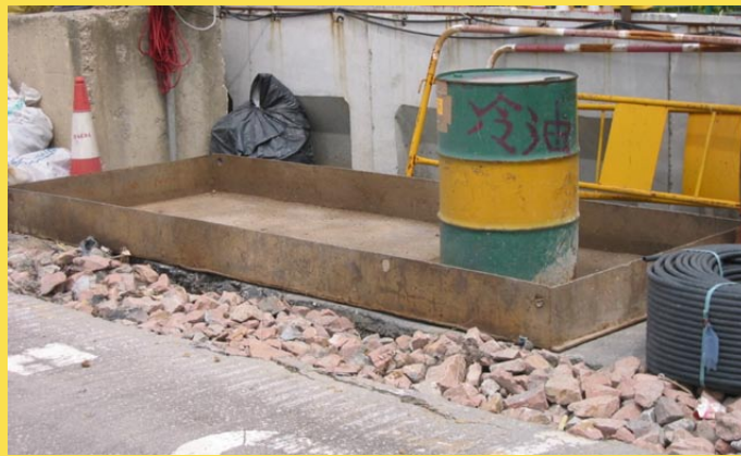
Drip tray underneath containers to prevent spillage
