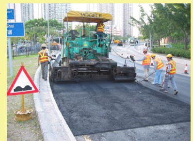
Laying of asphalt pavement with RAP material
