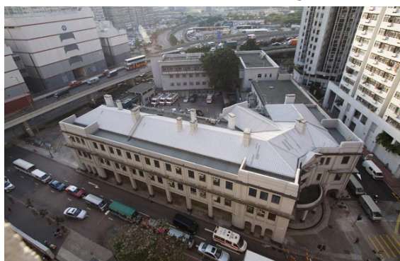
Old Wing of Police Station: Identified as a building of high significance
