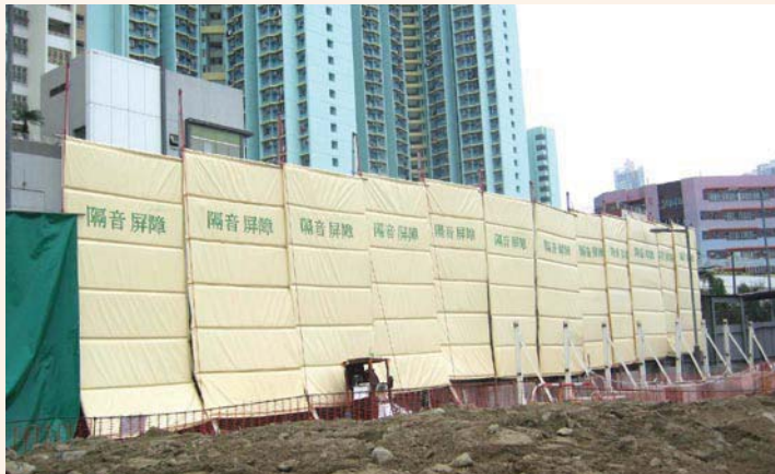
Temporary Noise Barrier
