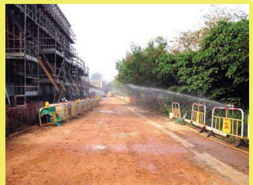
Installing sprinkler system along haul roads
