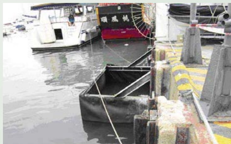
Installation of silt screen around seawater intake
