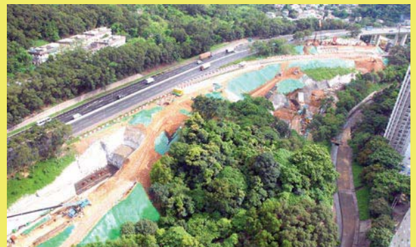
Covering the temporary excavation surface with shortcrete or tarpaulin
