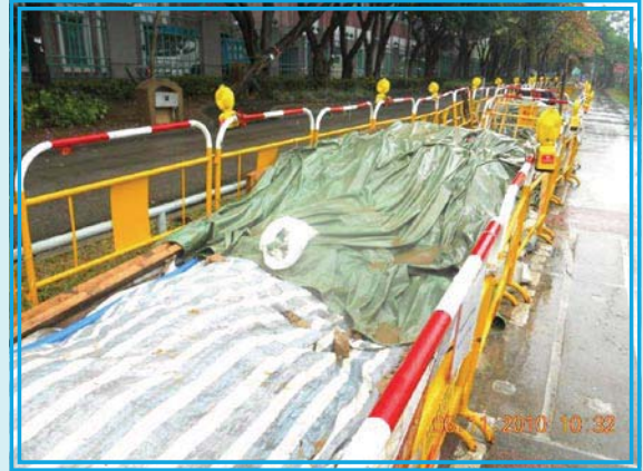
Small scale covering by tarpaulin sheet in work front
