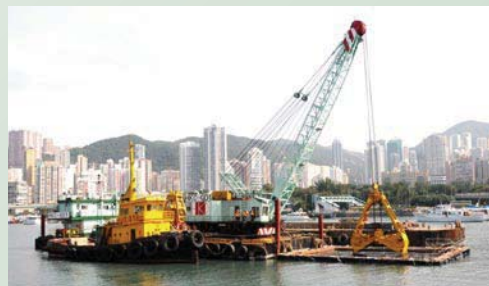
Deployment of silt curtain around dredging area
