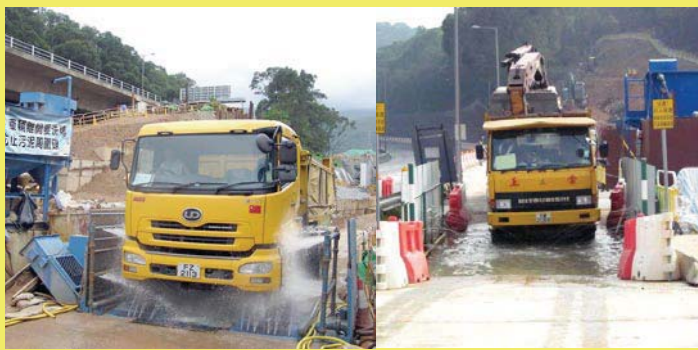
Installation of wastewater treatment unit (Aquasep) for wheel washing purpose
