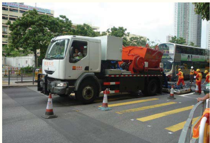
Field trial of hot-in-place recycling using larger size thermal patcher
