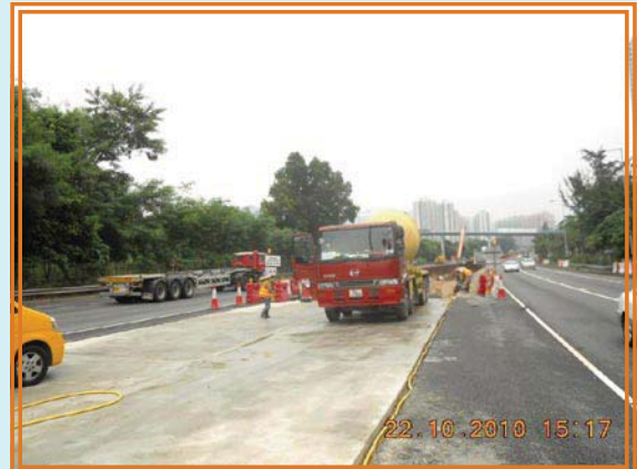
Paved area for the regular movement of vehicle
