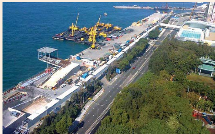
Construction of the Conveyor Belt System
