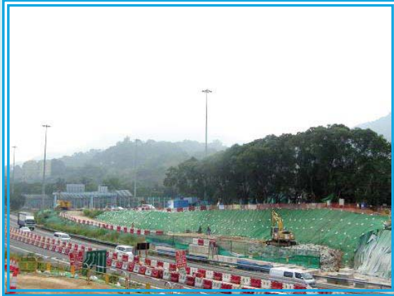
Large scale covering by tarpaulin sheet on exposed slope
