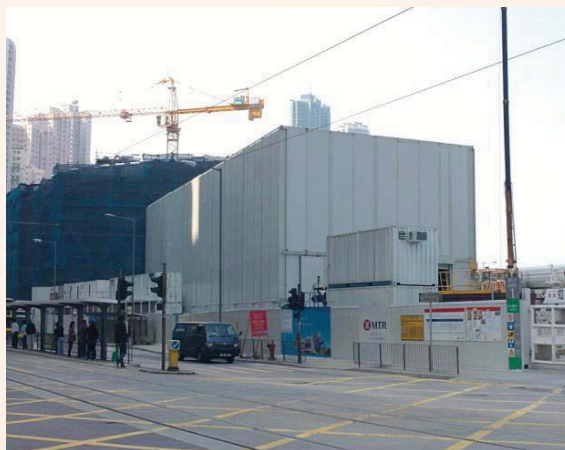
Noise Enclosure at Kennedy Town Praya
