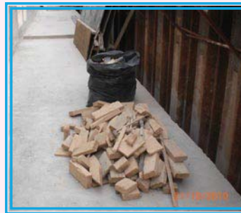
On-site sorting of construction and demolition material
