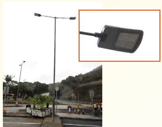
LED Road Lights
