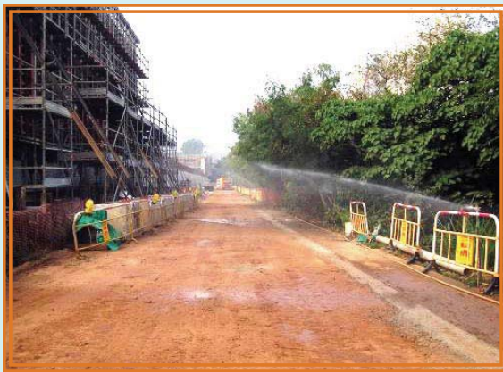
Installation of water sprinkler system to water temporary haul roads
