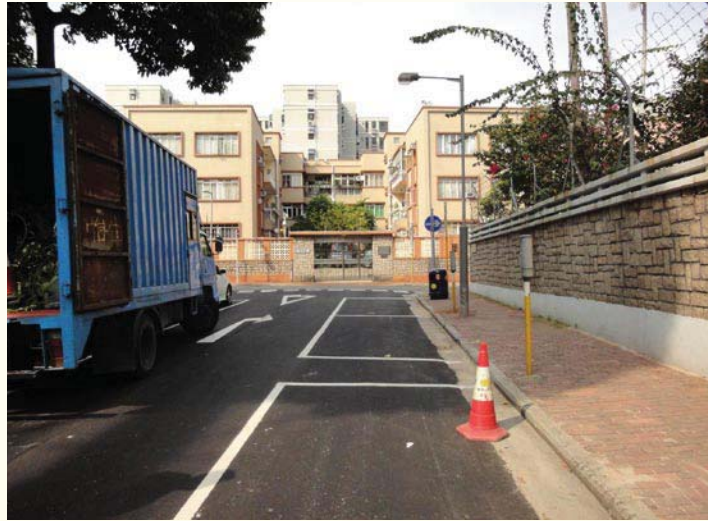
Trial site using 30% RAP at Verbena Road
