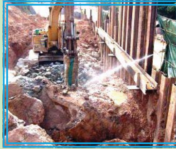
Temporary acoustic enclosure on concrete breakers during concrete/rock breaking up works
