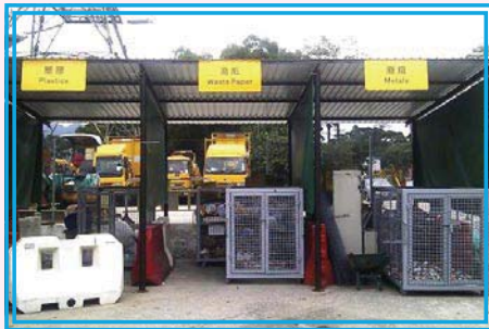
On-site sorting facilities and waste storage area
