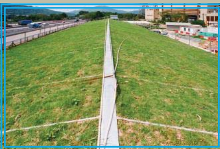
Grass roofing of site office
