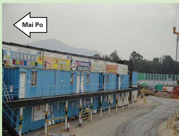
Double layer containers strategically positioned to serve as noise barrier
