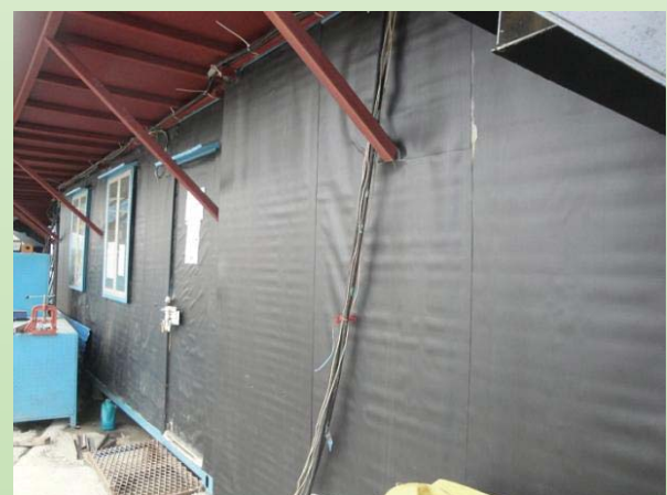
Noise absorption material applied to the container for maximum noise mitigation
