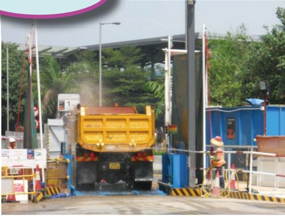
On-site automated wheel washing facility
