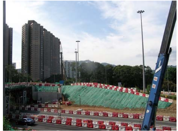
Tarpaulin sheet on exposed slope to prevent dust generation
