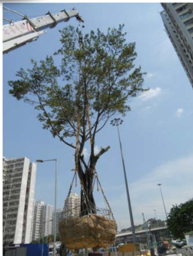
Tree transplanting with wire mesh net for rootball protection
