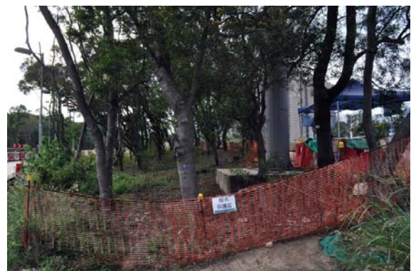
Retained trees are fenced off
