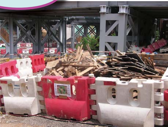
On-site sorting of waste timber for recycling
