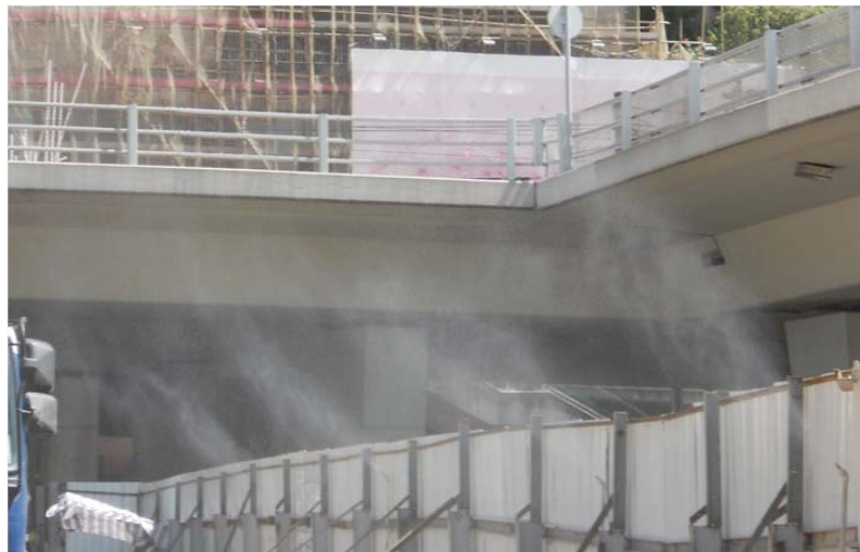
Water spraying system along site hoarding for dust suppression
