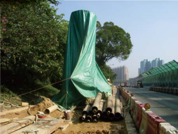
Drilling rigs covered with tarpaulin sheets
