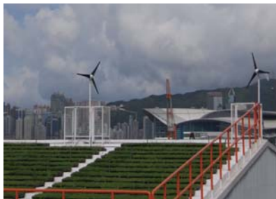
Wind turbines for electricity generation
