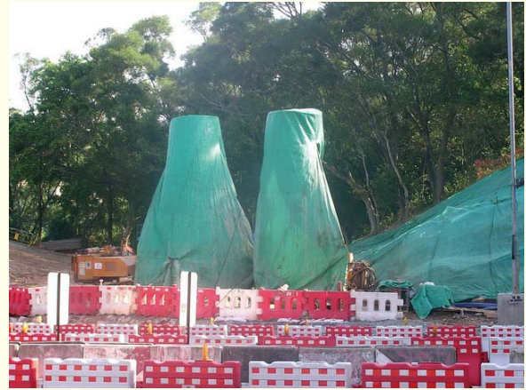
Drilling rigs covered by tarpaulin sheets
