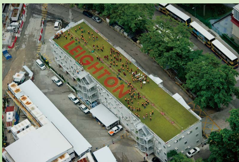
Green roof provided for Ocean Park Station site office
