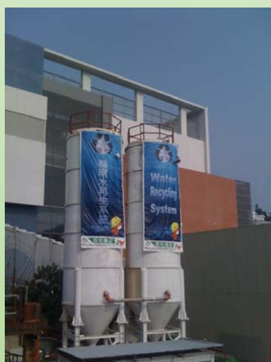
Construction run-offs treatment and reuse at Nam Fung Tunnel Portal
