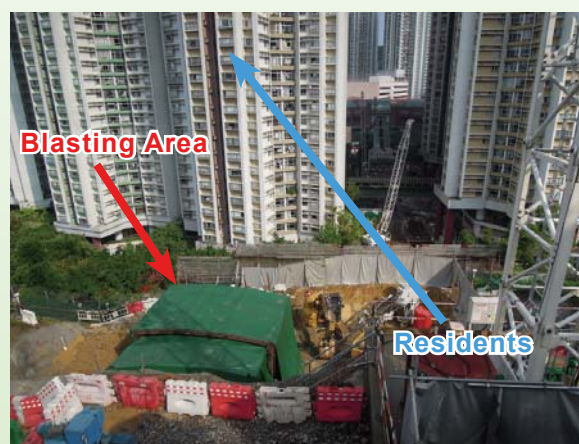
Open blasting for construction of Wong Chuk Hang Depot and South Horizon End Plant Building
