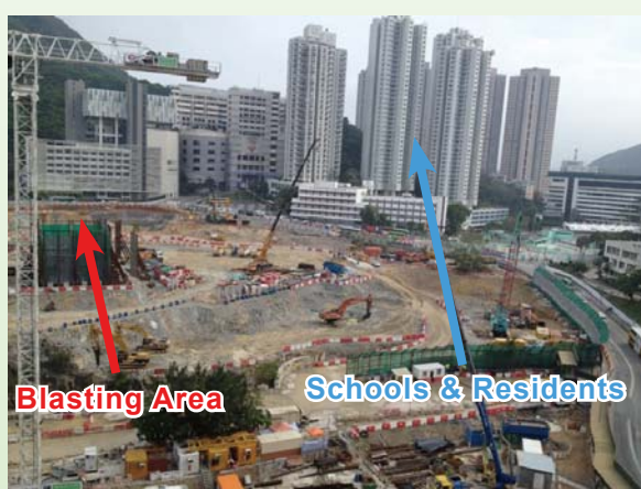
Open blasting for construction of Wong Chuk Hang Depot and South Horizon End Plant Building
