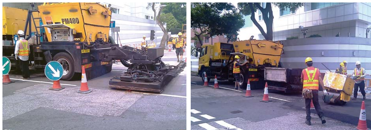
Thermal Patcher in operation
