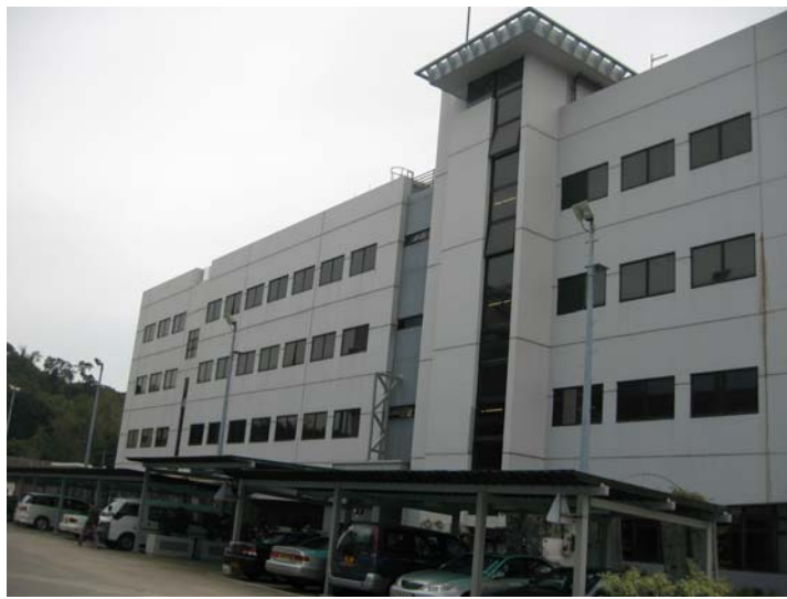
Reflective Cellulose Films on GD's Administration Building
