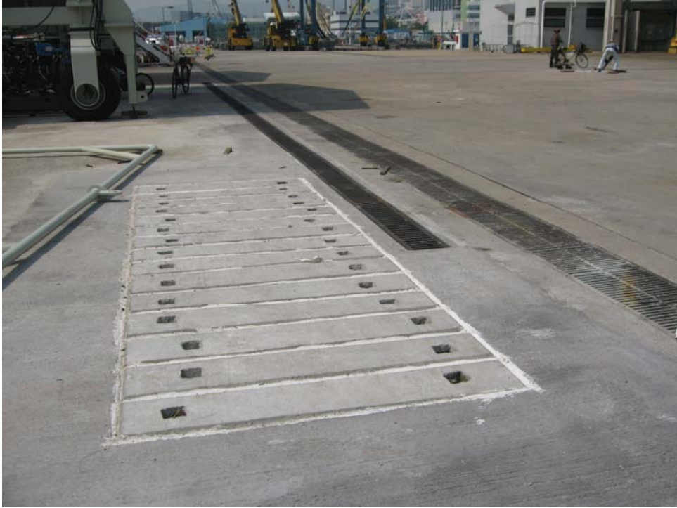
Extension of Sewage Treatment System in Open Yard in GD
