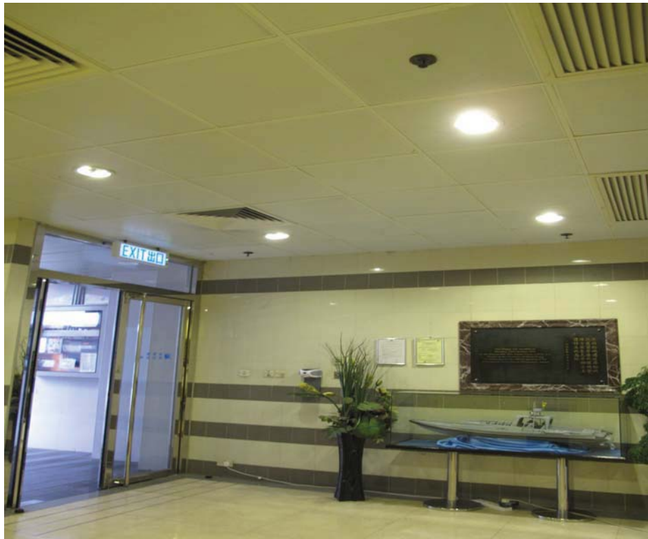
LED lighting in Administration Building of GD
