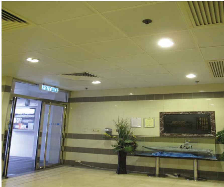
LED lighting in Administration Building of GD
