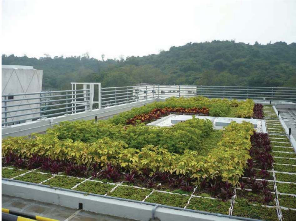
Green Roof at the Administration Building in GD
