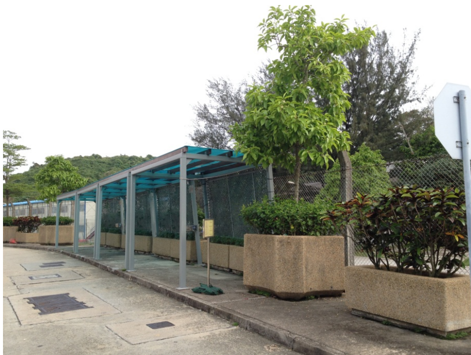
Additional Flower Pots Erected Alongside Coach Waiting Area in GD
