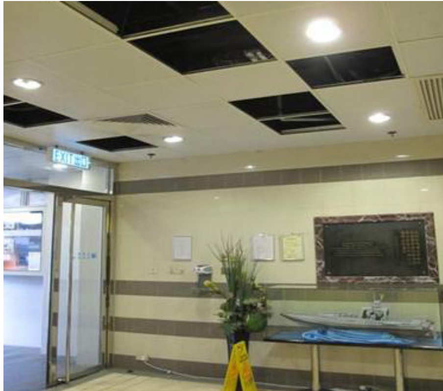
Replacement of Lighting by LED Energy Saving Lights
