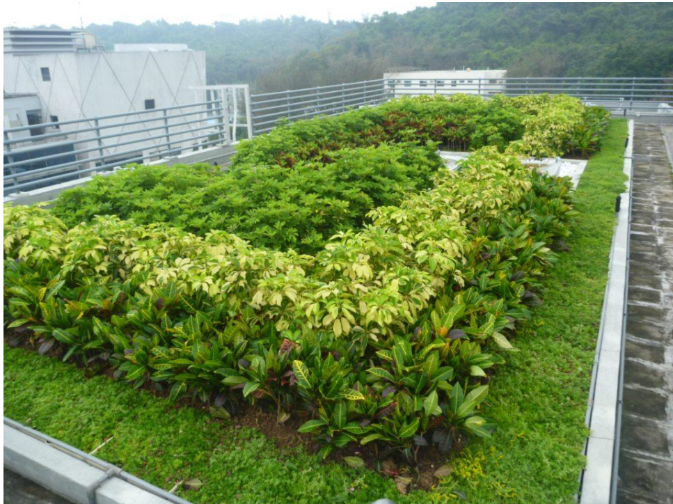
Green Roof on Block A, GD
