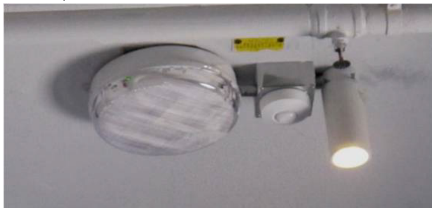
Installation of Proximity Switches for Lighting
