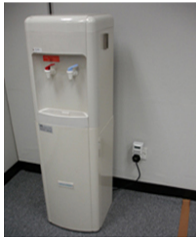
7-day timer switches are installed at distilled water dispensers to automatically switch off the dispensers after office hours.
