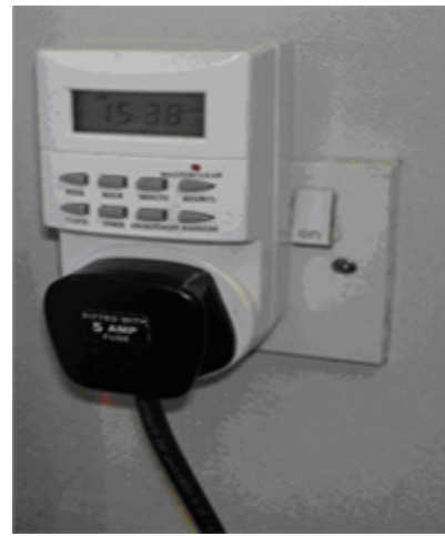
7-day timer switches are installed at distilled water dispensers to automatically switch off the dispensers after office hours.
