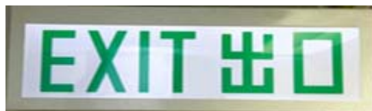
Fluorescent tube exit signs are replaced by LED type to reduce power consumption.
