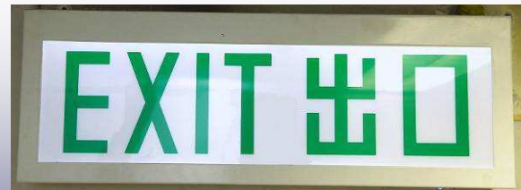
Fluorescent tube exit signs are replaced by LED type to reduce power consumption.
